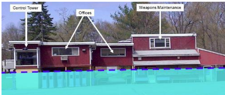
(Photograph courtesy of the Dep't of Administrative Services Construction Services)
