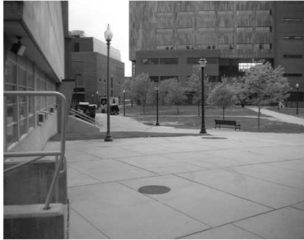
Looking west toward Pharmacy/Biology Building and Central Utility Plant
