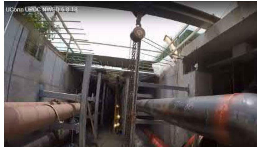
Figure 3.13. Example of Utility Tunnel Interior (Gant Utility Tunnel June 8, 2018) Source: https://youtu.be/MKlvm5cVAzo
