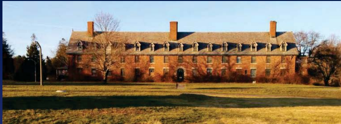
Nurses' Residence, a.k.a. Employees Building
