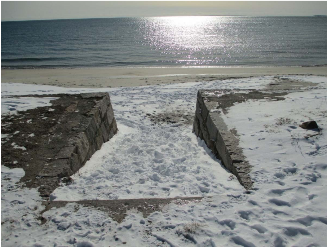
Photo 3-16. Stairway in seawall leading down to beach
