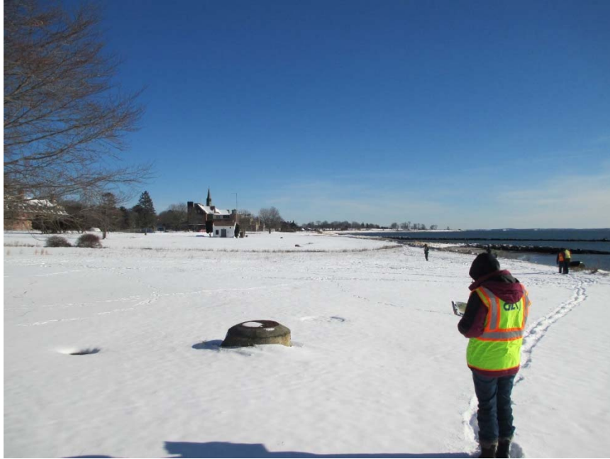
Photo 3-12. Elevated sewer manhole along easement
