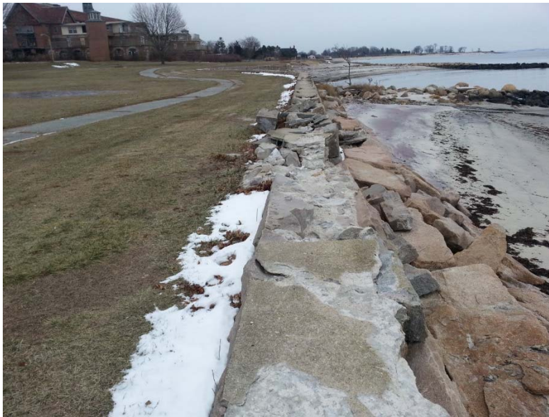
Photo 3-9. Easterly view along seawall at central cove
