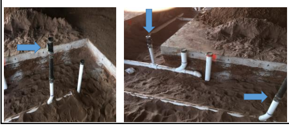
Examples of properly bedded piping and test tees.
