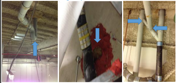
Plumbing inspections cont.
