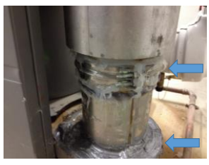
Direct vent boiler flue connection
