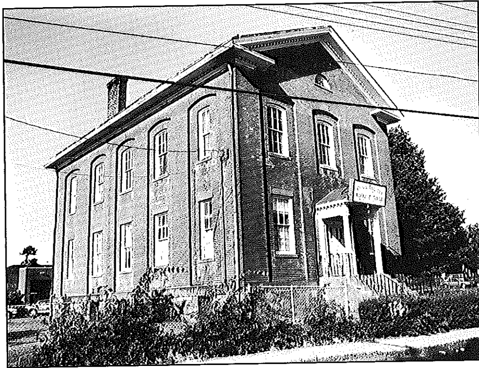
13. Goffe Street School, New Haven, 1864. View west.
