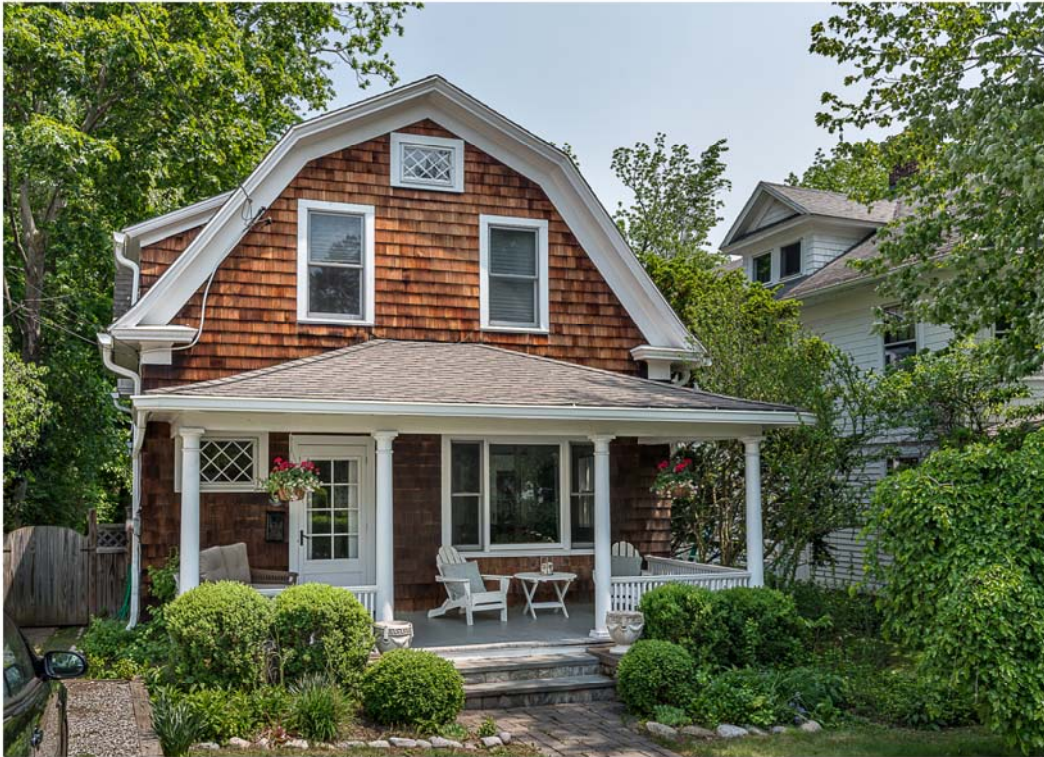
Photo 17. View north of 25 Lincoln Street showing facade.
