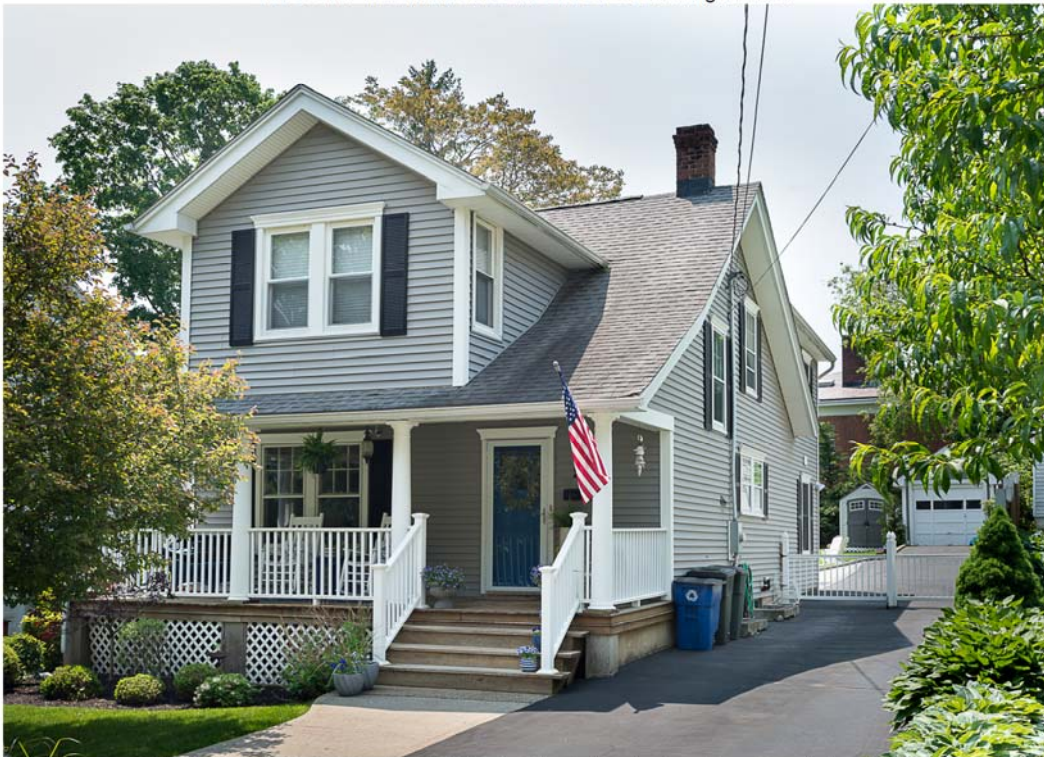
Photo 18. View southeast of 26 Lincoln Street showing facade and west elevation.
