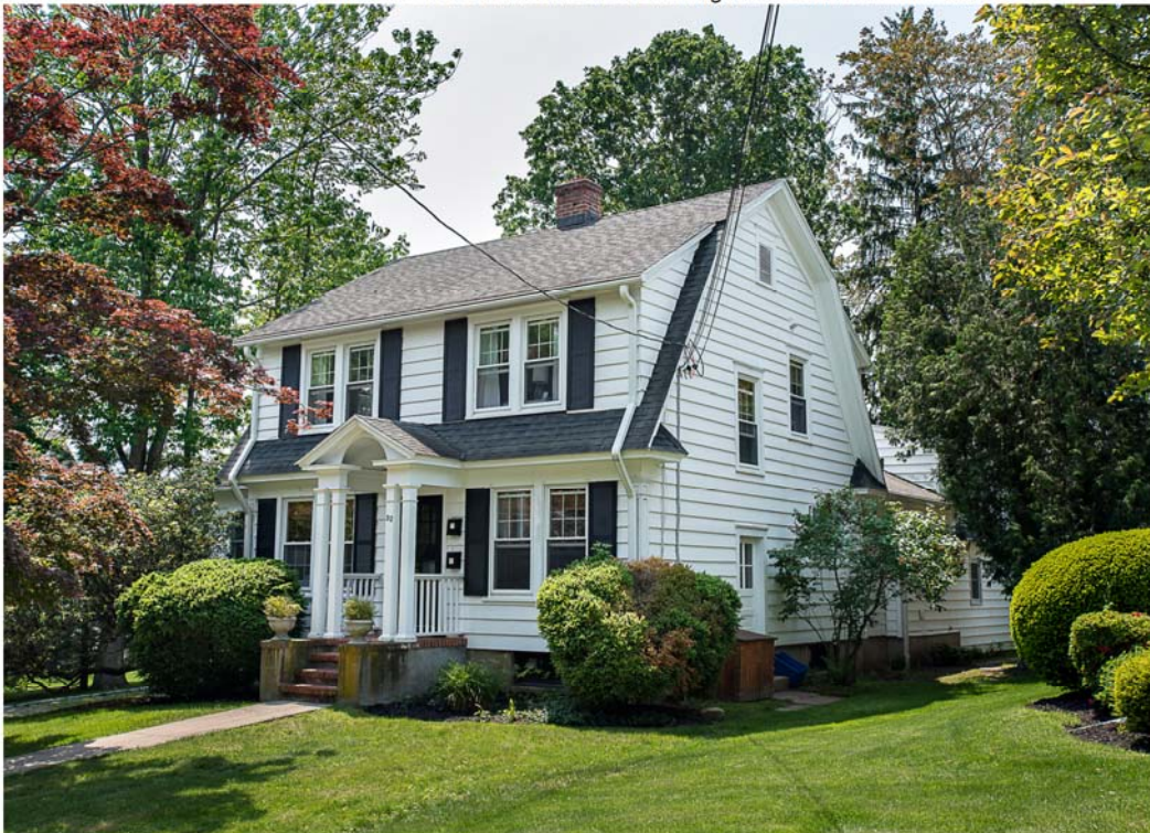
Photo 20. View southeast of 32 Lincoln Street showing facade and west elevation.
