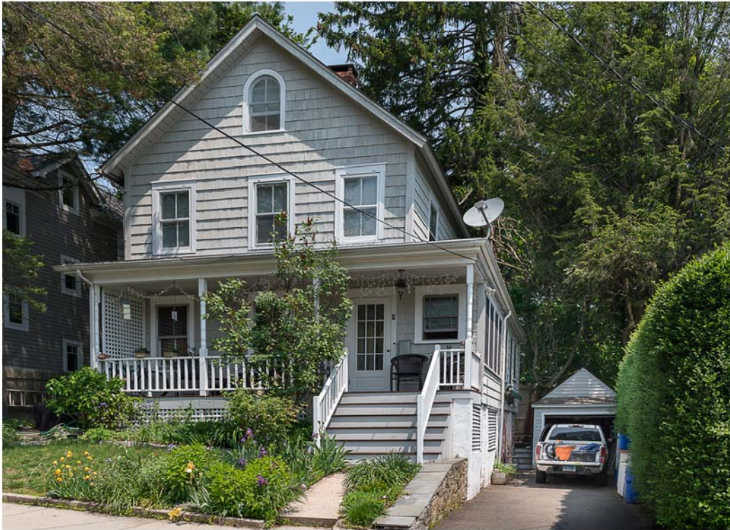
Photo 11. View north of 7 Lincoln Street showing facade.
