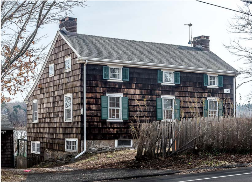
Photo 1. 125 Riverside Avenue, view southeast showing north and west elevations.
