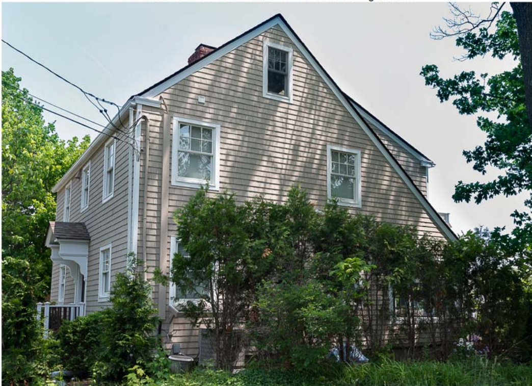
Photo 30 View north of 75 Riverside Avenue showing facade and south elevation..
