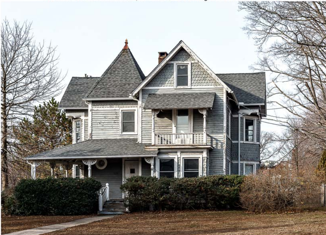
Photo 40. 136 Riverside Avenue, view southwest showing facade.
