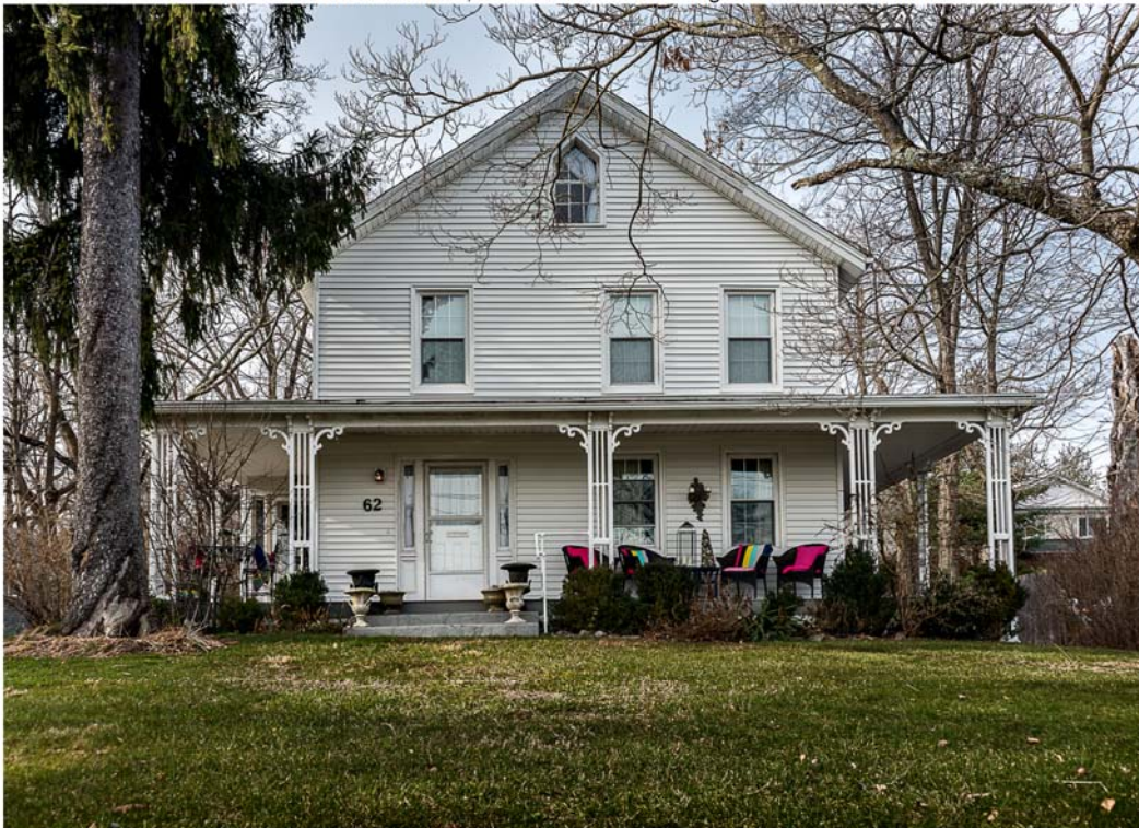
Photo 28. 62 Riverside Avenue, view east showing facade.
