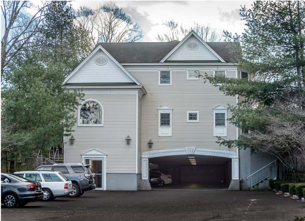
Photo 7. 20 Cross Street, view south showing facade.
