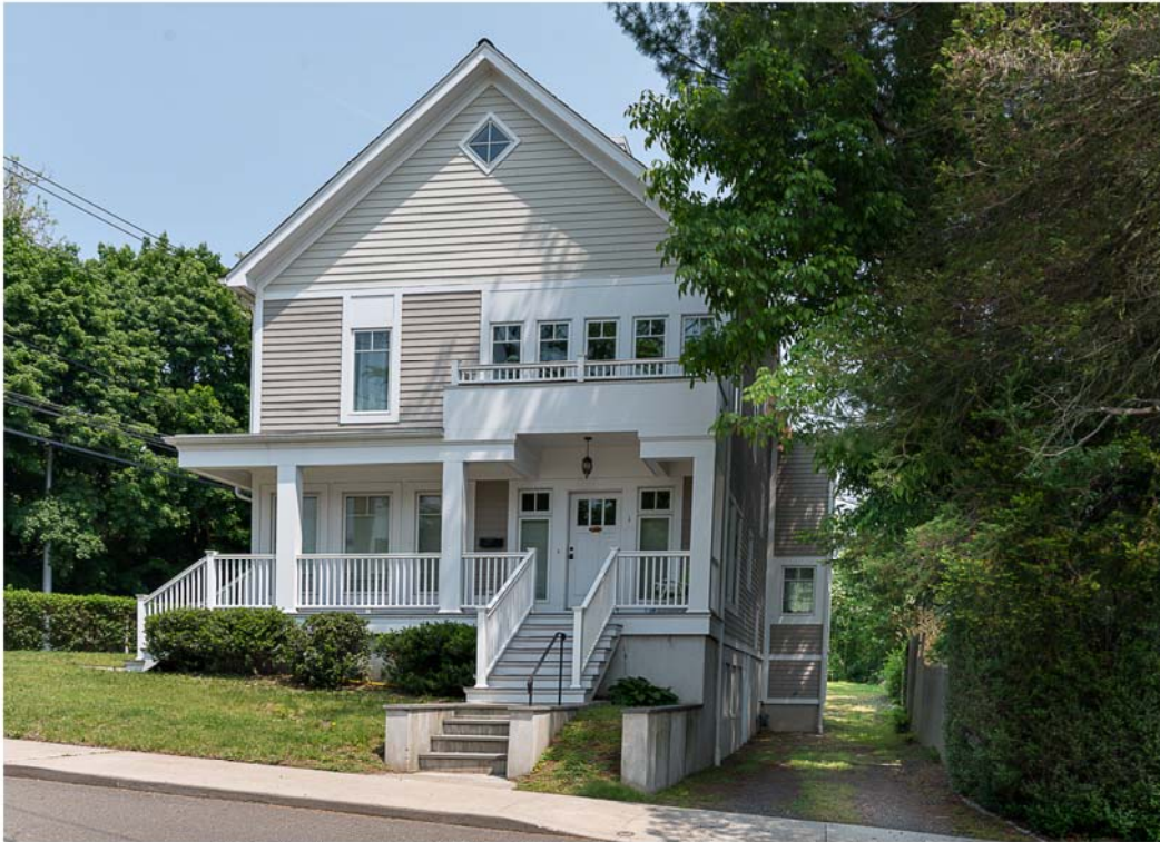
Photo 9. View north of 1 Lincoln Street showing facade and east elevation.
