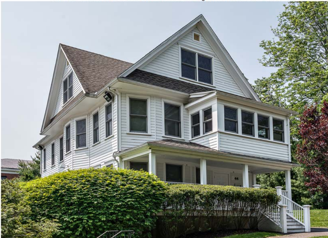
Photo 22. View southwest of 44 Lincoln Street showing east elevation and facade.
