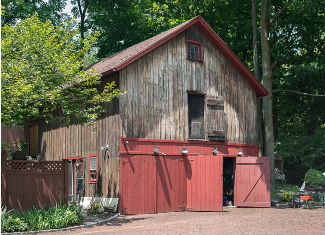
Photo 41. View northwest of barn to the west of 82 Riverside Avenue showing south elevation and facade.
