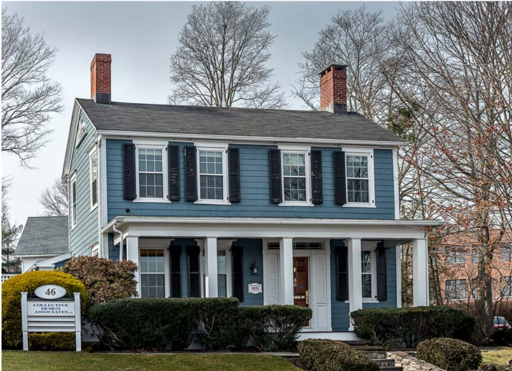
Photo 25. 46 Riverside Avenue, view northwest showing south elevation and facade
