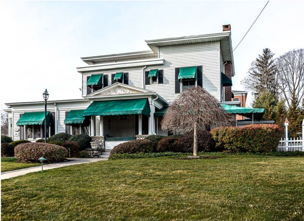
Photo 35. Former 114 Riverside Avenue,, view west showing facade.
