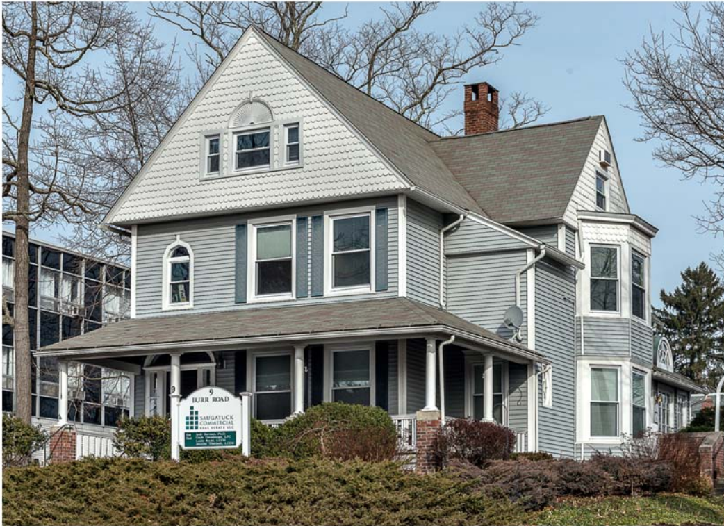
Photo 3. 9 Burr Road, view northwest showing facade and east elevation.
