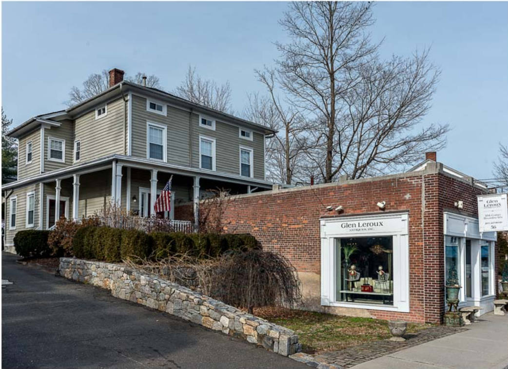
Photo 27. 56 Riverside Avenue, view northwest showing south elevation and facade.
