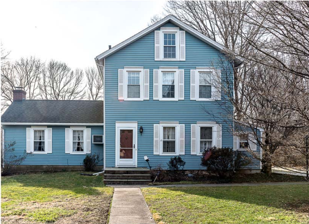
Photo 5. 18 Burr Road, view south showing facade.
