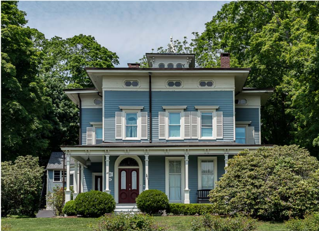
Photo 29. View west of 68 Riverside Avenue showing facade.
