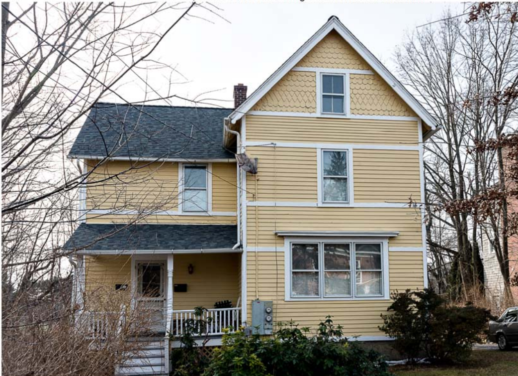
Photo 4. 16 Burr Road, view south showing facade.
