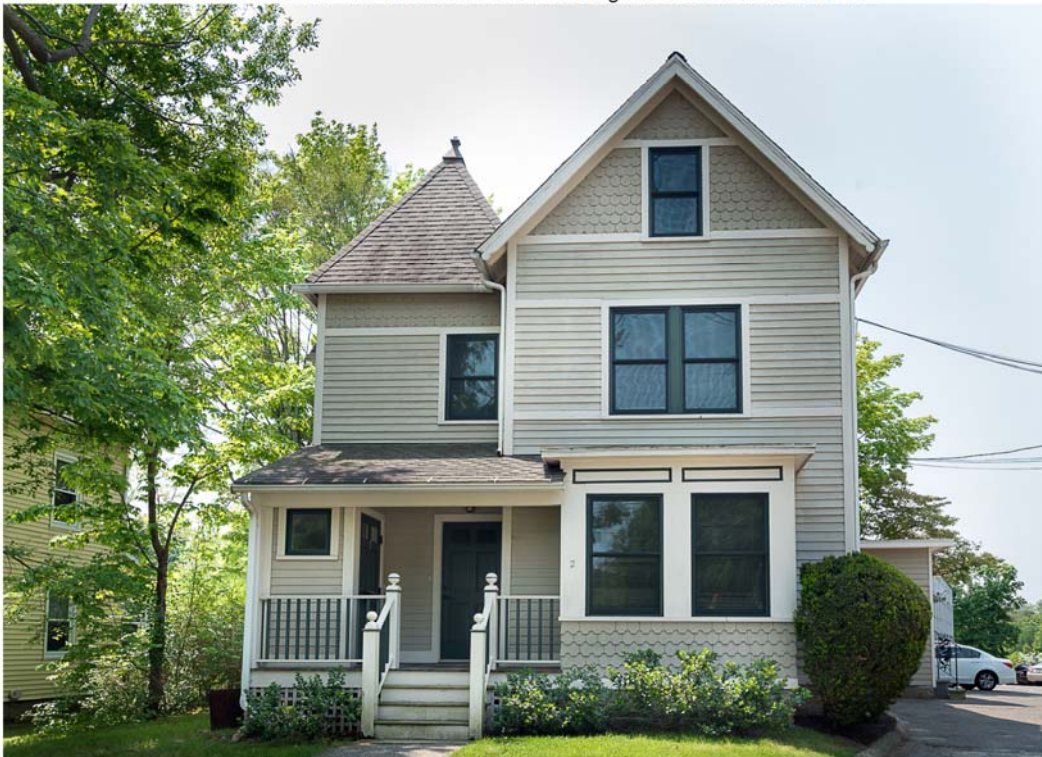
Photo 10. View south of 2 Lincoln Street showing facade.
