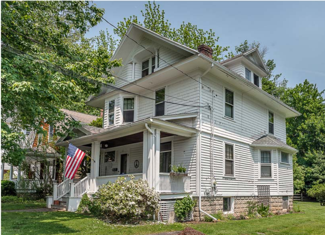
Photo 19. View northwest of 31 Lincoln Street showing facade and east elevation.
