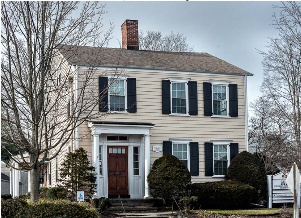
Photo 26. 50 Riverside Avenue, view northwest showing south elevation and facade.
