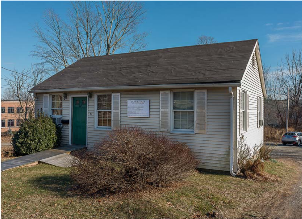
Photo 23. View northeast of 57 Post Road West showing facade and south elevation.
