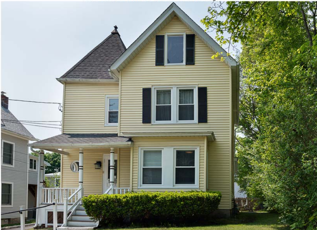
Photo 12. View south of 8 Lincoln Street showing facade.
