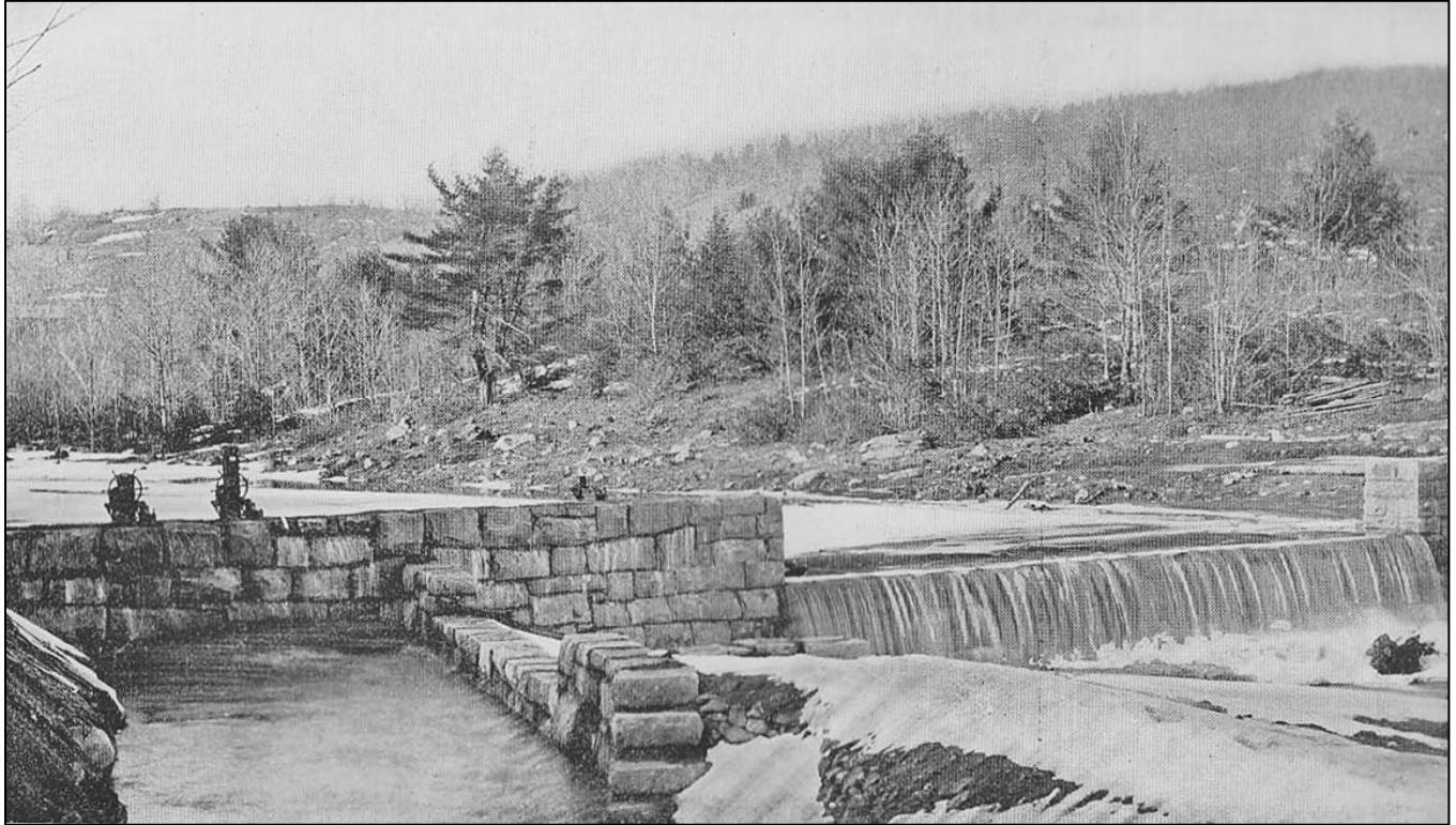
Figure 4: Mad River Canal and Mad River Dam, ca. 1894 (Winsted, CT, Water Improvement Committee 1896).
