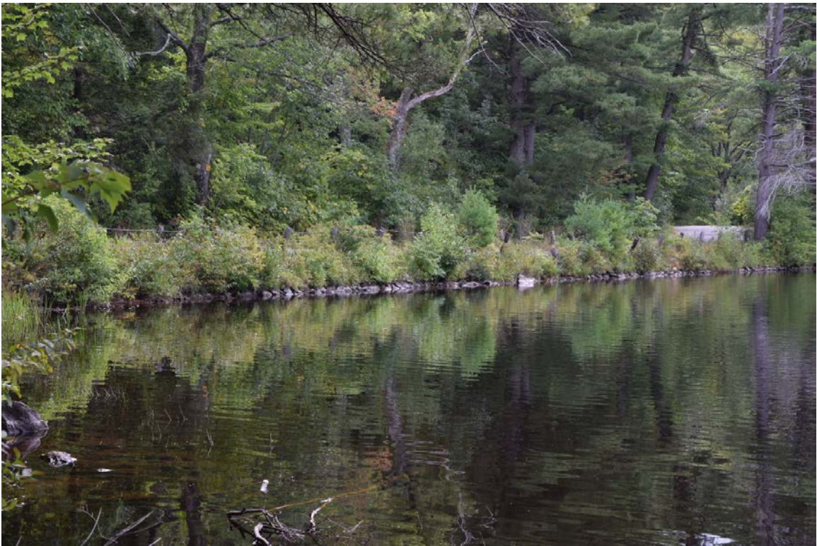
Photo 9. Rugg Brook North Dike, looking southeast.
