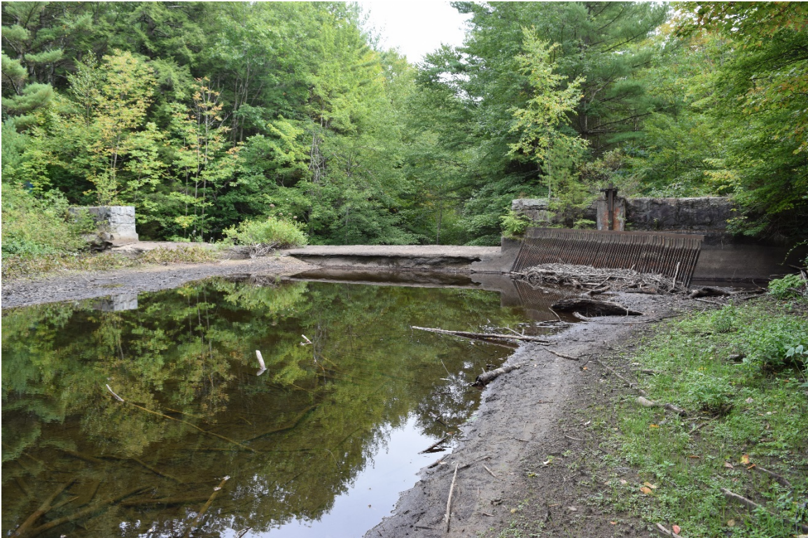
Photo 1. Mad River Diversion Dam, looking east.
