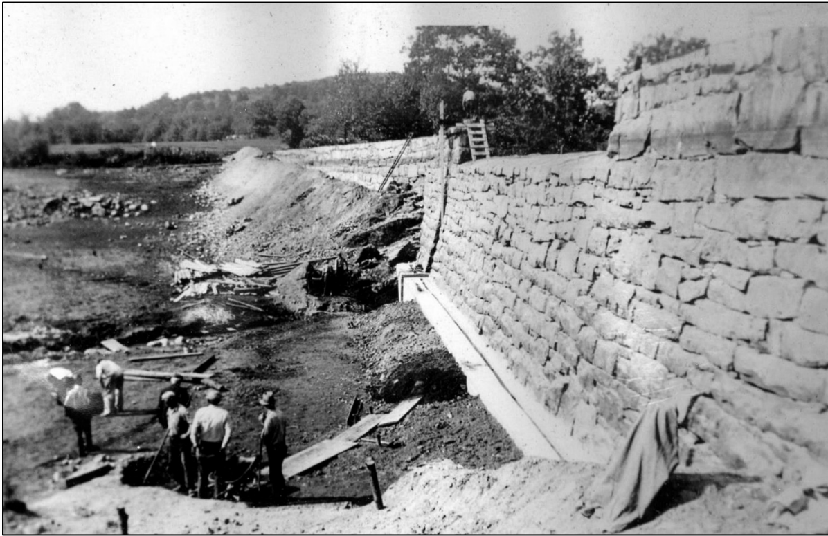
Figure 6: Upstream side of Rugg Brook Dam, ca. 1935, before the addition of the concrete liner (courtesy Dave Battista, Lenard Engineering, Winsted, CT).
