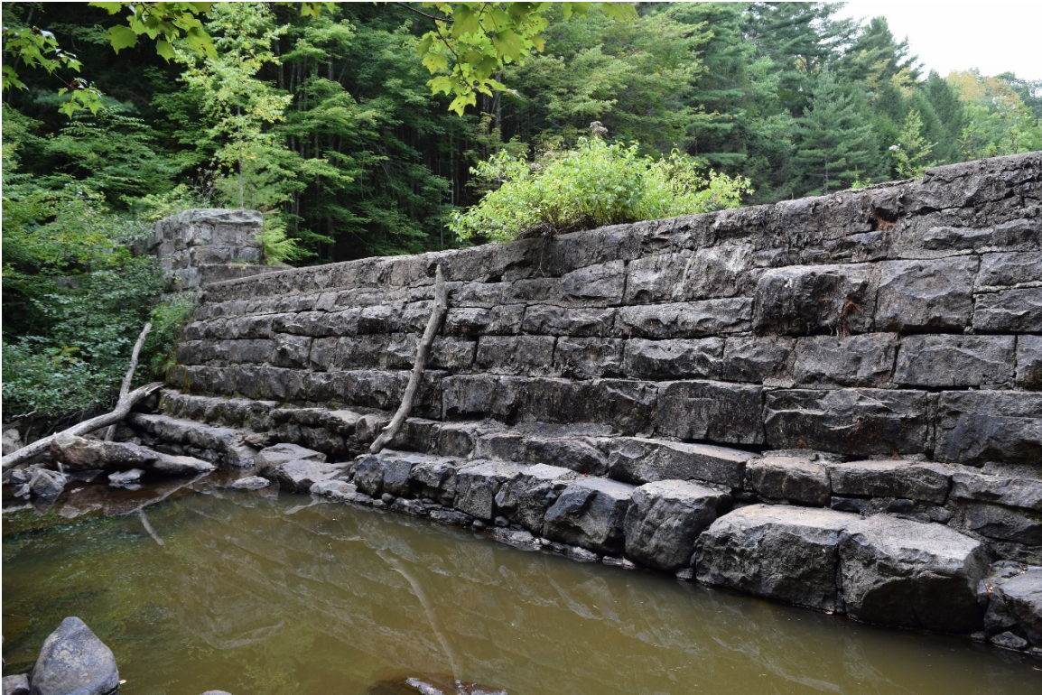
Photo 2. Mad River Diversion Dam, looking southwest.
