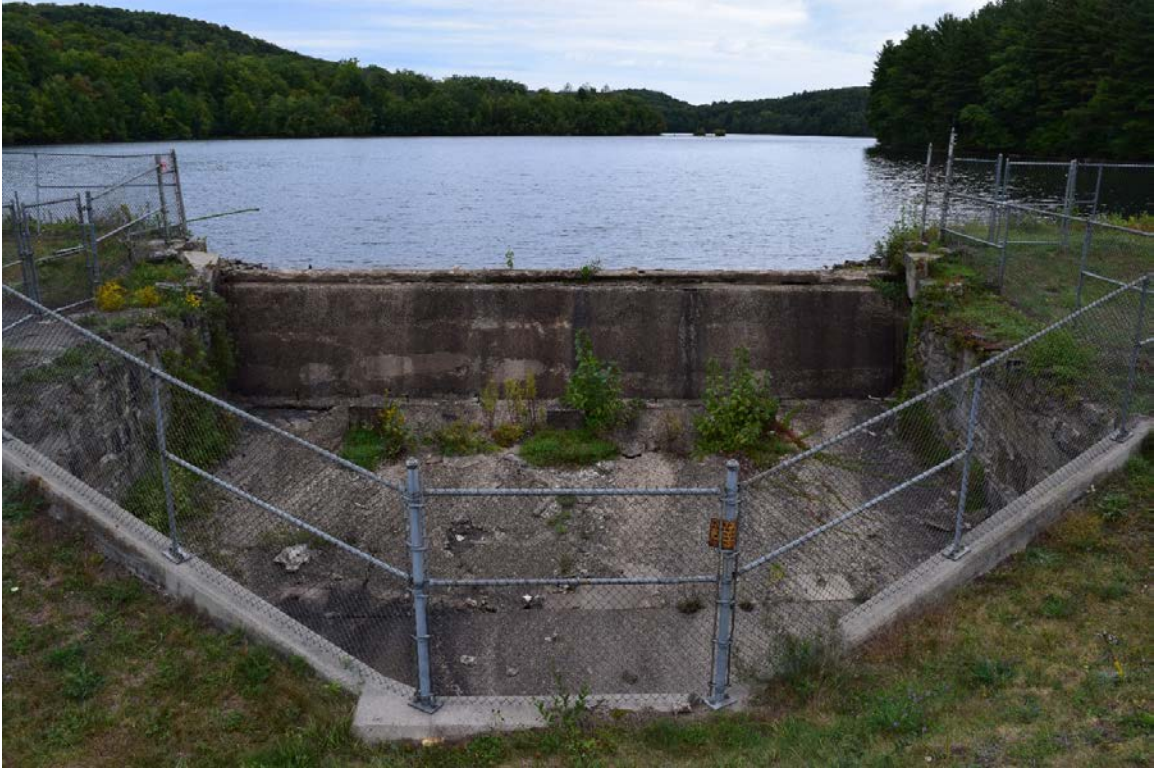
Photo 16. Crystal Lake Dam spillway, looking north.
