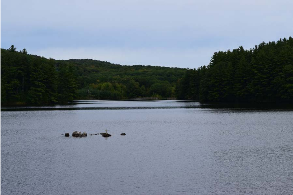
Photo 6. Rugg Brook Reservoir and Dam, looking north.
