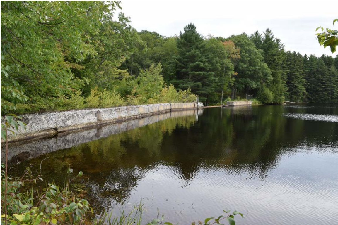
Photo 7. Rugg Brook Reservoir Dam, looking east.
