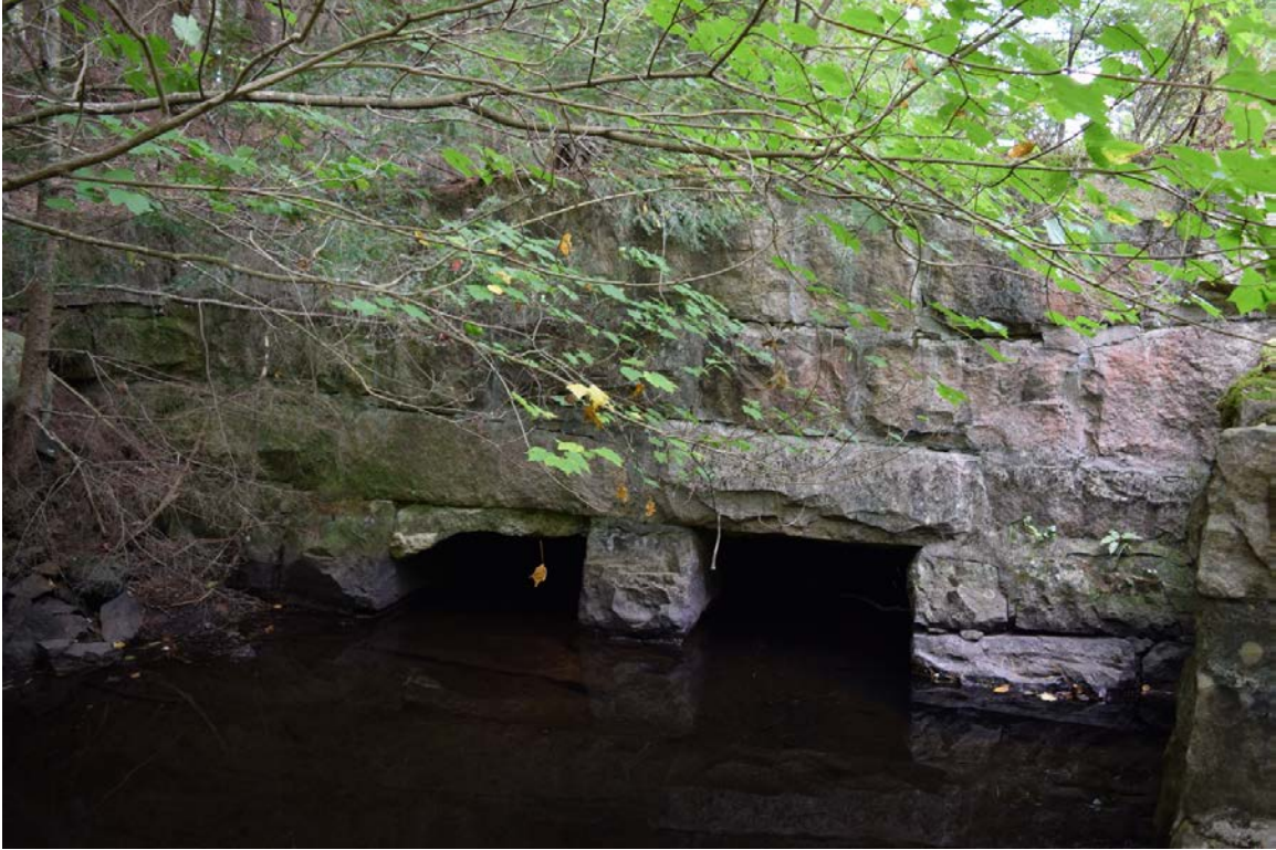
Photo 4. Mad River Diversion Canal, looking west.
