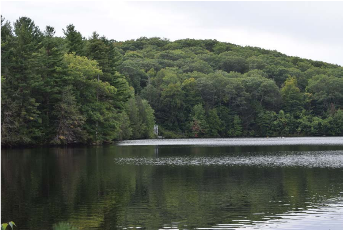
Photo 11. Gilbert Tunnel Inlet Works, looking south.
