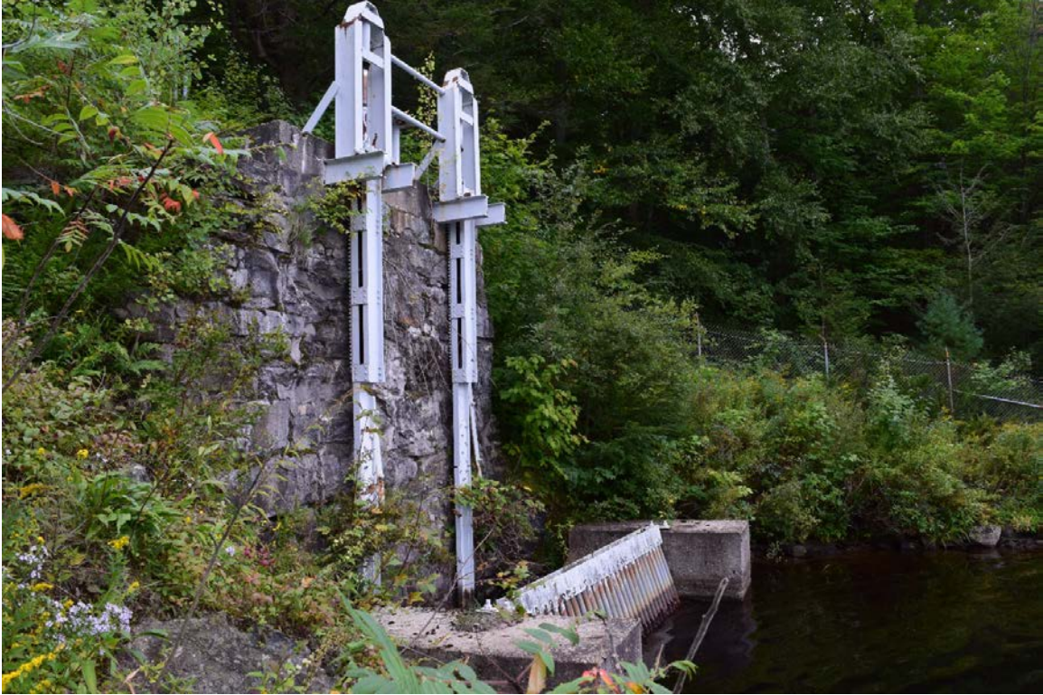
Photo 12. Gilbert Tunnel Works, looking southwest.
