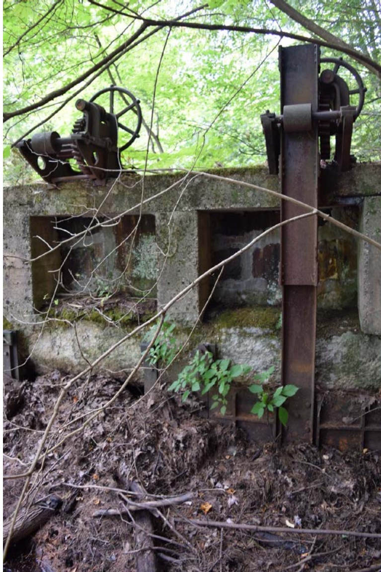
Photo 3. Mad River Diversion Canal Gates, looking east.
