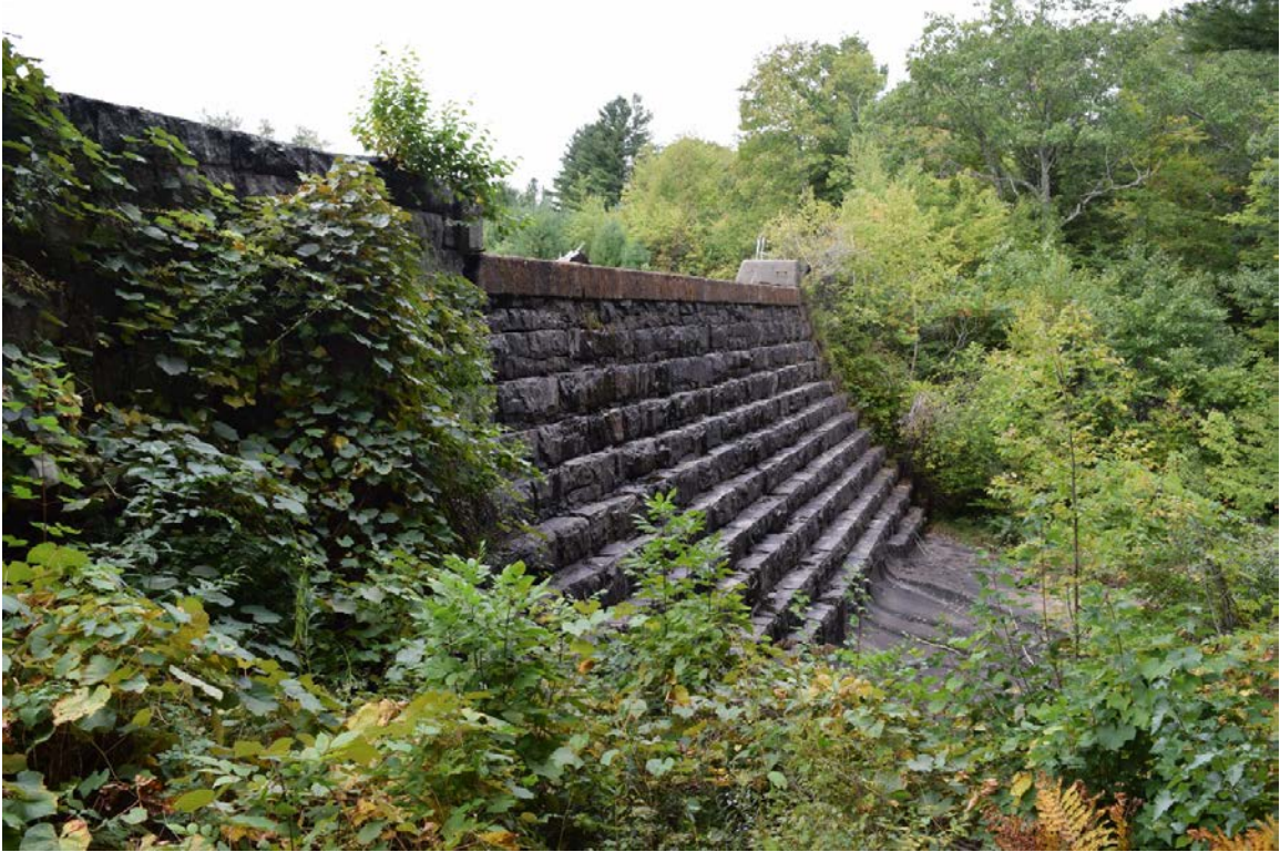
Photo 8. Rugg Brook Reservoir Dam, looking west.
