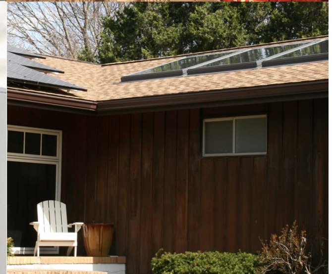
Photo by Mitsubishi Electric
