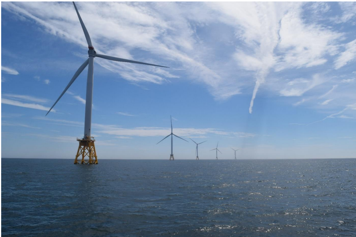
Figure 6-2. Although offshore wind energy turbines are unlikely to occur in Long Island Sound, new facilities and infrastructure could enter Long Island Sound. The Block Island Wind farm shows the potential for new renewable energy infrastructure through the Northeast. Photo Credit: Emily Hall
