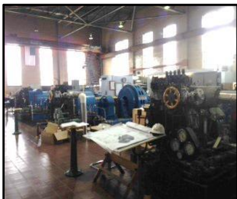
Figure 6: Connecticut Valley Hospital
