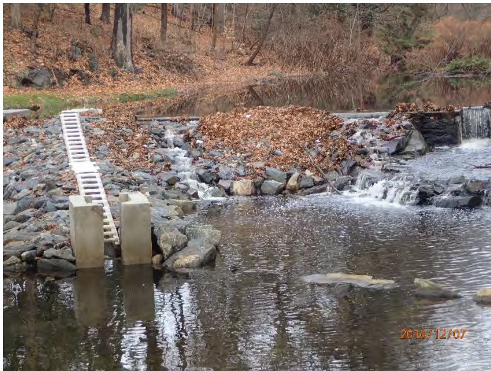
The Upper Pond Fishway is at the head-of-tide on the Goodwives River.
