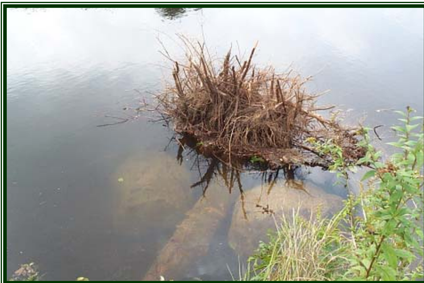
Final placement view of tree and rootwad. Boulders help to secure rootwad in place.
