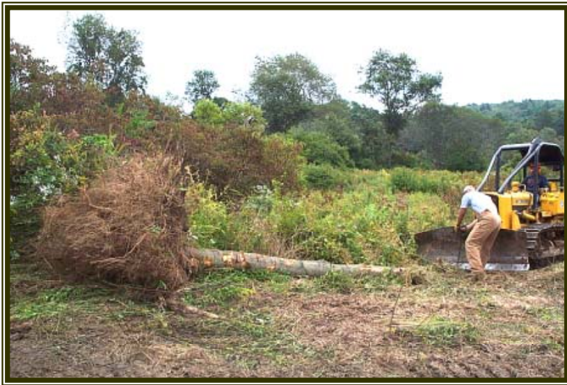
Excavated tree and rootwad being transported to the river's edge for installation.
