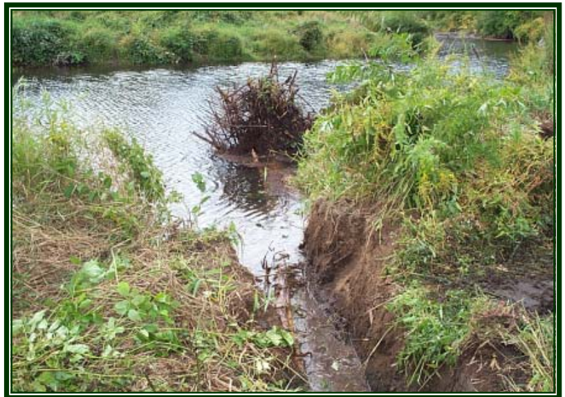
Tree and rootwad installed into excavated trench.
