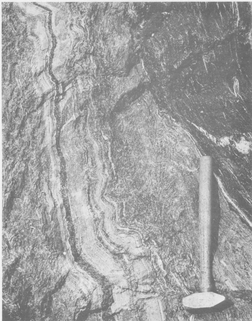
Fig. 8. Interlayered granulitic gneiss, schist, and amphibolite in Hartland Formation unit I in the railroad cut immediately south of East Litchfield. Scale given by 14-in. hammer.
