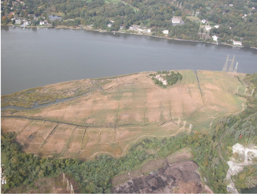
Power Line Marsh in Milford – Aerial by Roger Wolfe 10/02/12
