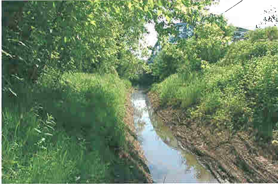
CT DOT Stormwater Drainage abutting Rt. 202 to south
