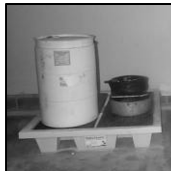
Proper waste storage-- closed, labeled drum stored inside with secondary containment
