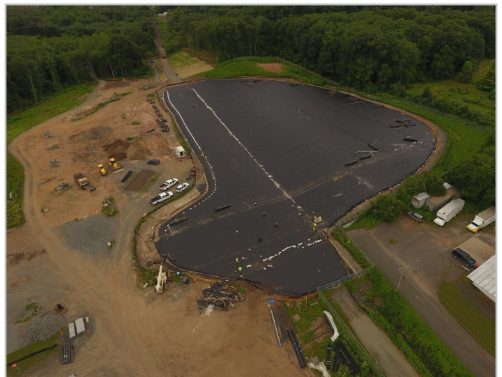
Figure 4 – Construction of cap in former Operations Area in progress (July 2017)
