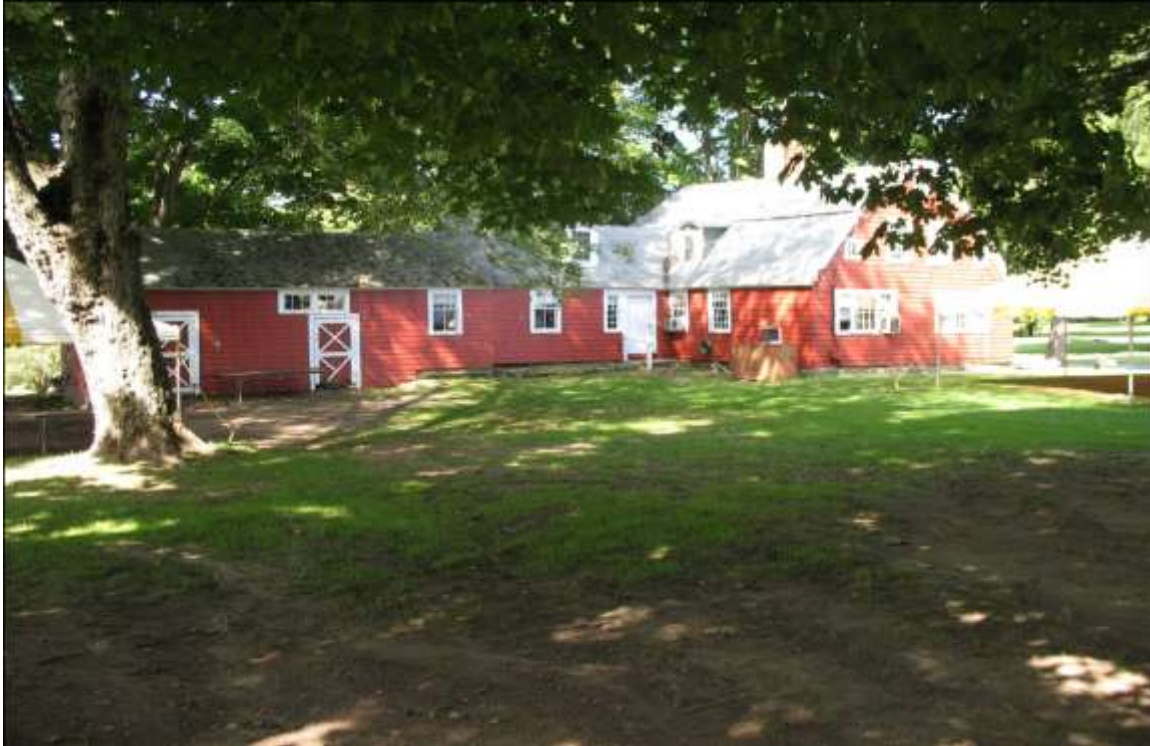
Picture 1. Toll House (Building #82) This structure is DEEP's highest priority for preservation and re-use.
