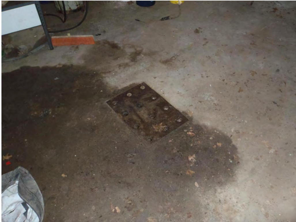
Photo 4-10 - AOC-08 (Maintenance Garage Floor Drain)
