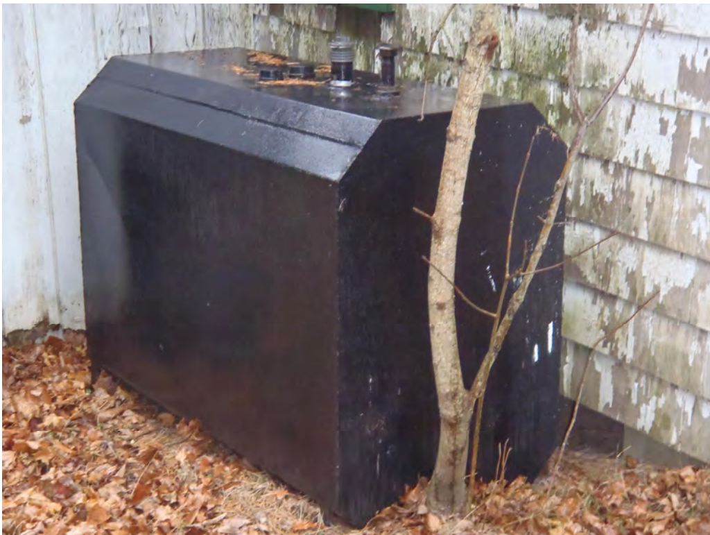
Photo 4-1 – AOC-01 (Example AST)
