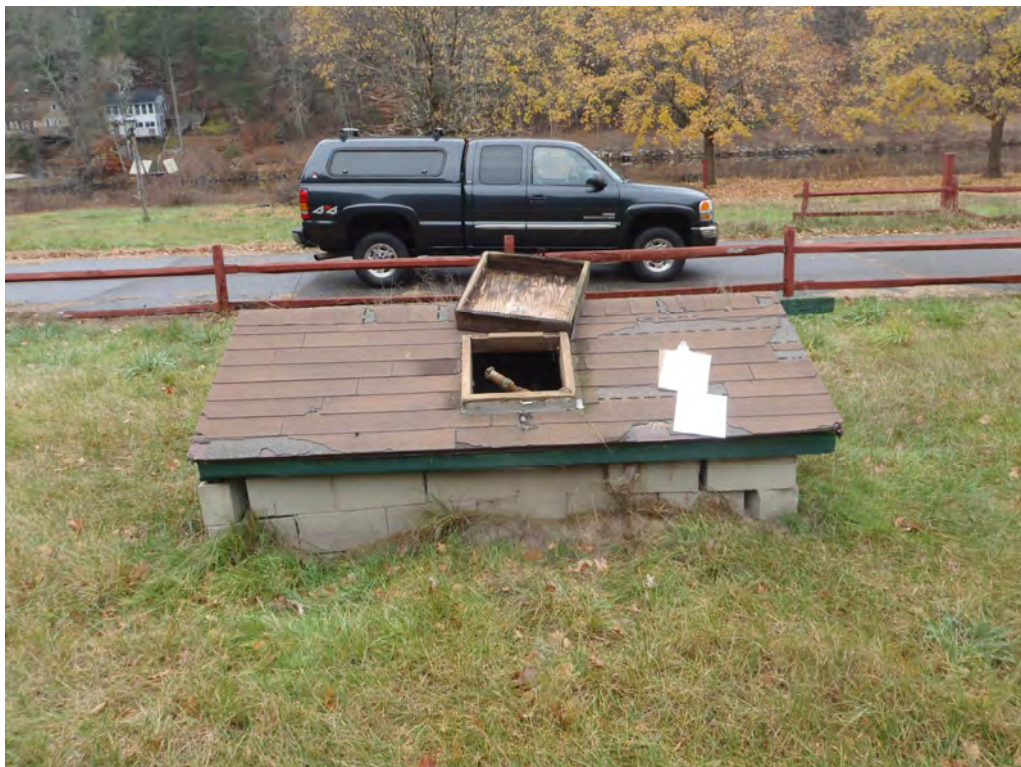
Photo 3-7 – Septic Pumping Wetwell
