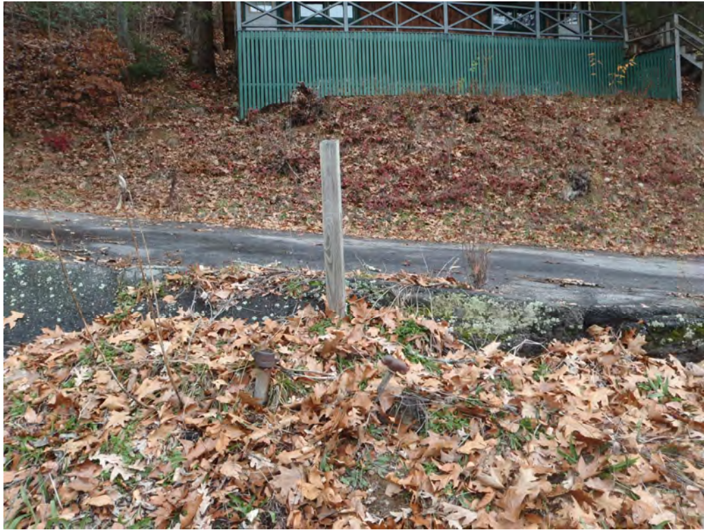
Photo 4-4 - AOC-05 (Suspected UST Vent Pipe)
