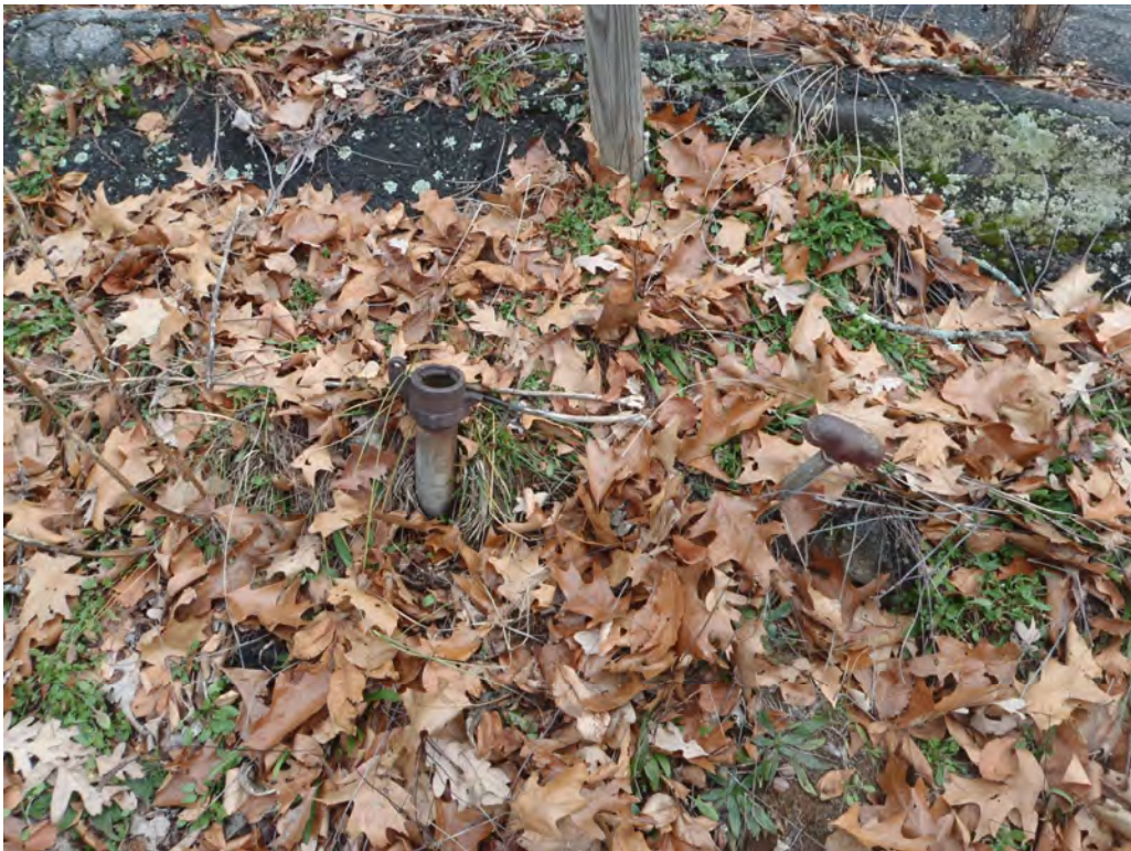
Photo 4-3 – AOC-04 (Suspected UST Vent Pipe)
