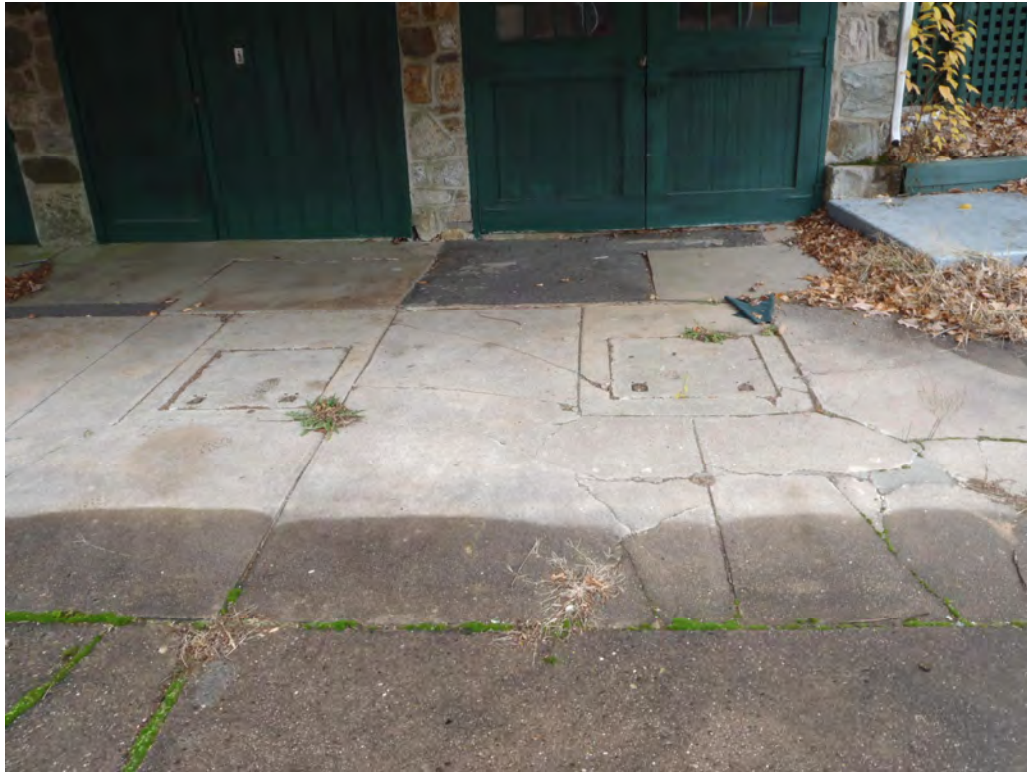
Photo 4-6 - AOC-07 (Suspected UST)
