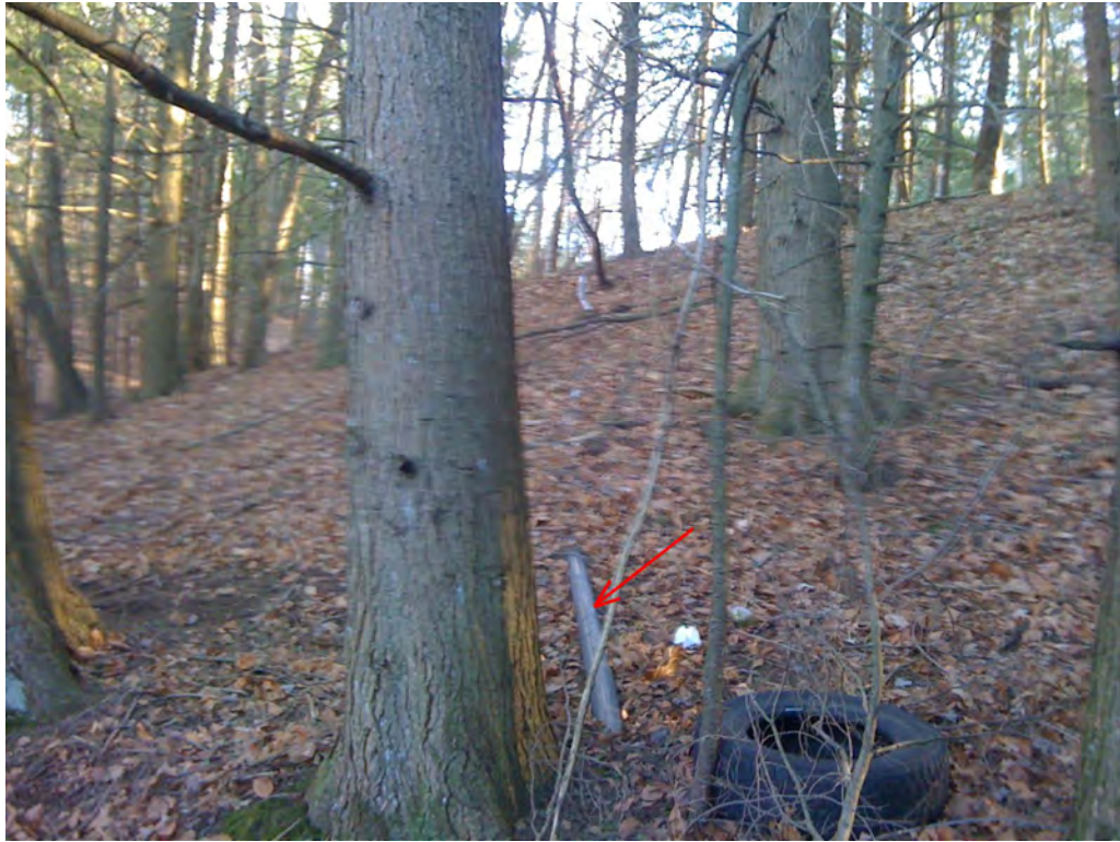
Photo 3-8 – Exposed Septic Forcemain
