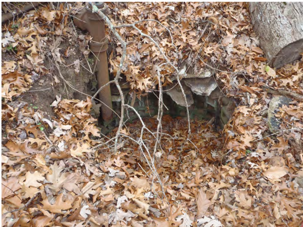
Photo 4-11 - AOC-10 (Sample Drywell)
