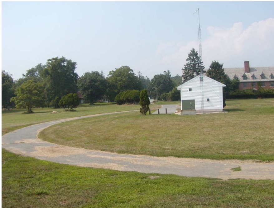
Photo 3-11. Municipal wastewater pump station
