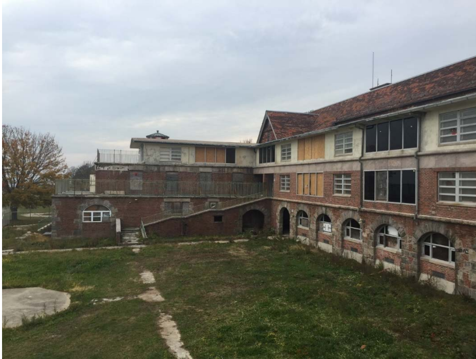
Photo 3-13. Terraces along Main Hospital, allowing multiple patients exposure to the outdoor elements and views of the ocean
