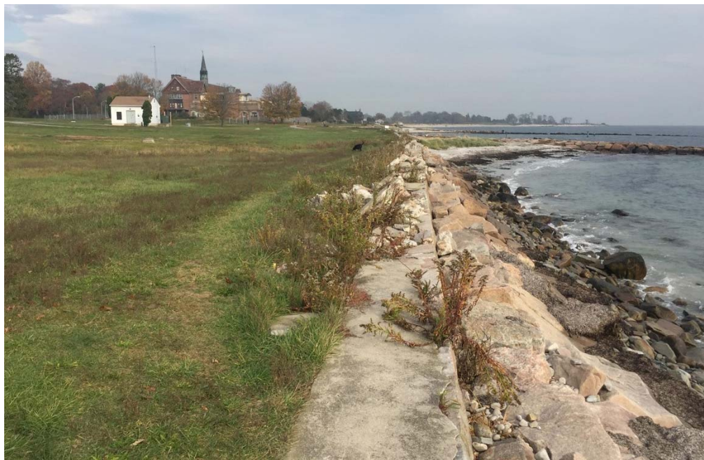
Photo 3-17. View of municipal pump house, former Main Hospital, lawns, seawall, and shoreline, facing east
