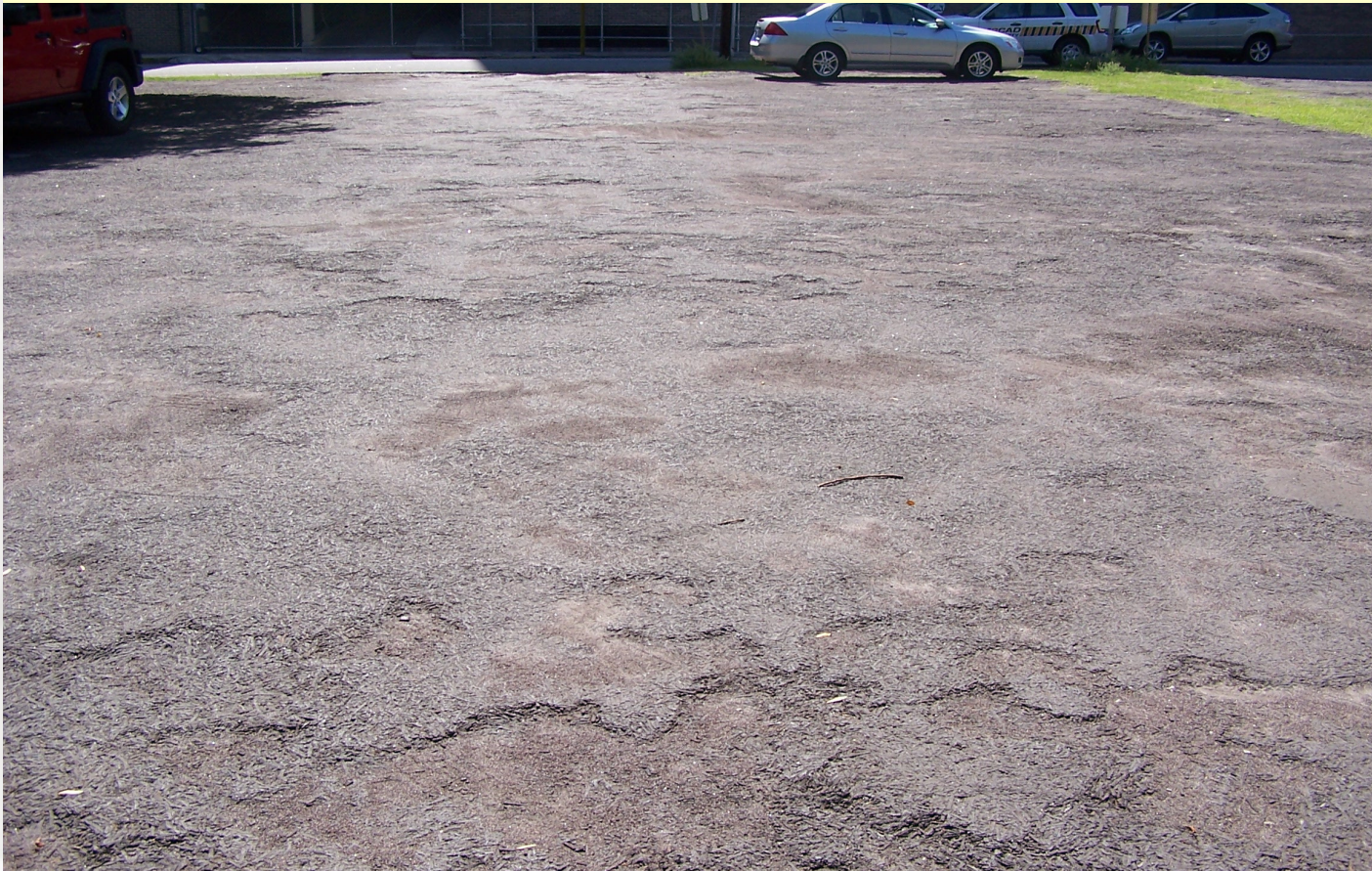
Parking Lot in Savannah, Georgia
