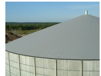
Biogas production optimized in percolate tank
