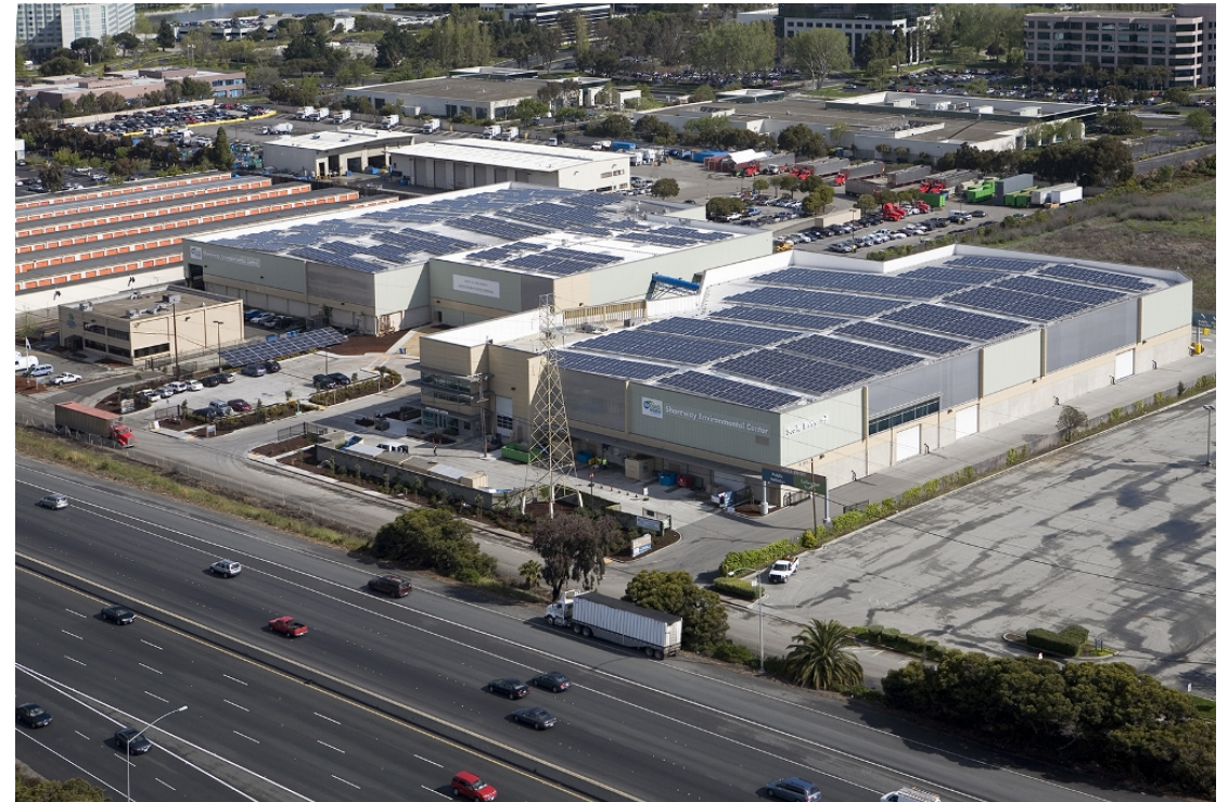
Recycling MRF and Transfer Station San Matteo, CA
