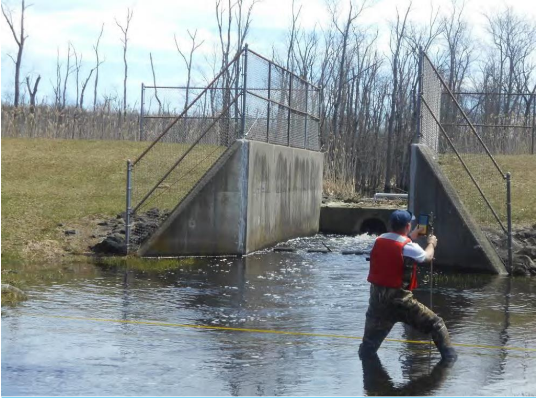
Figure 5 - Principal Spillway Outlet Looking Upstream
