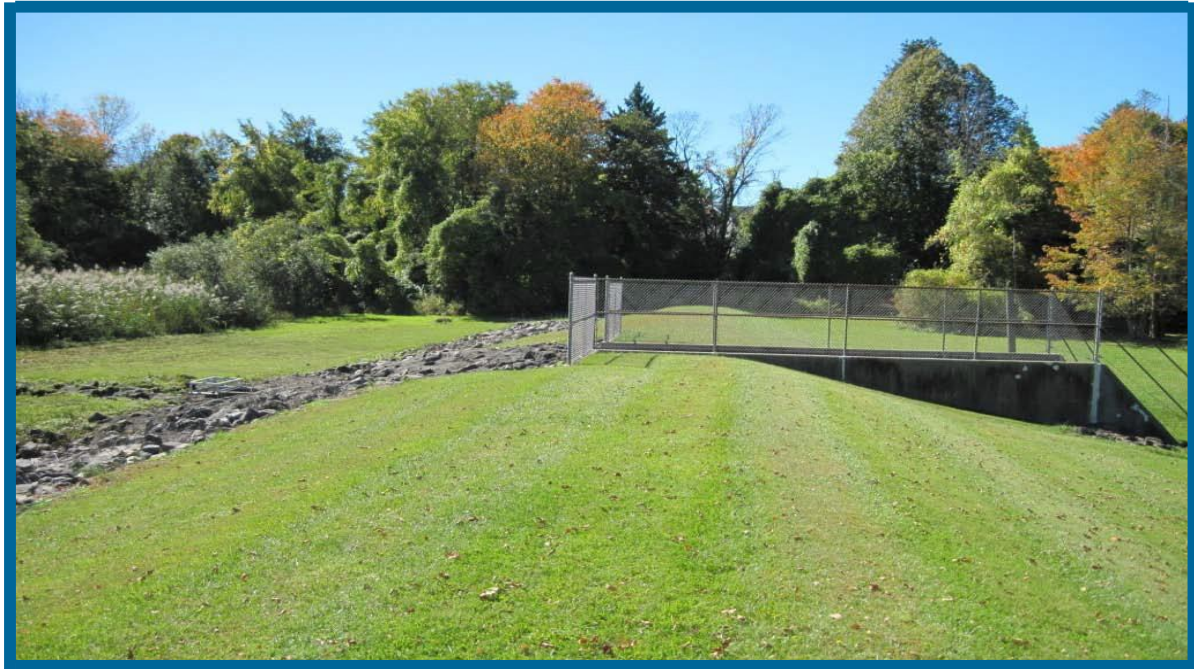
Figure 2 - Dam Embankment with Inlets to the Left
