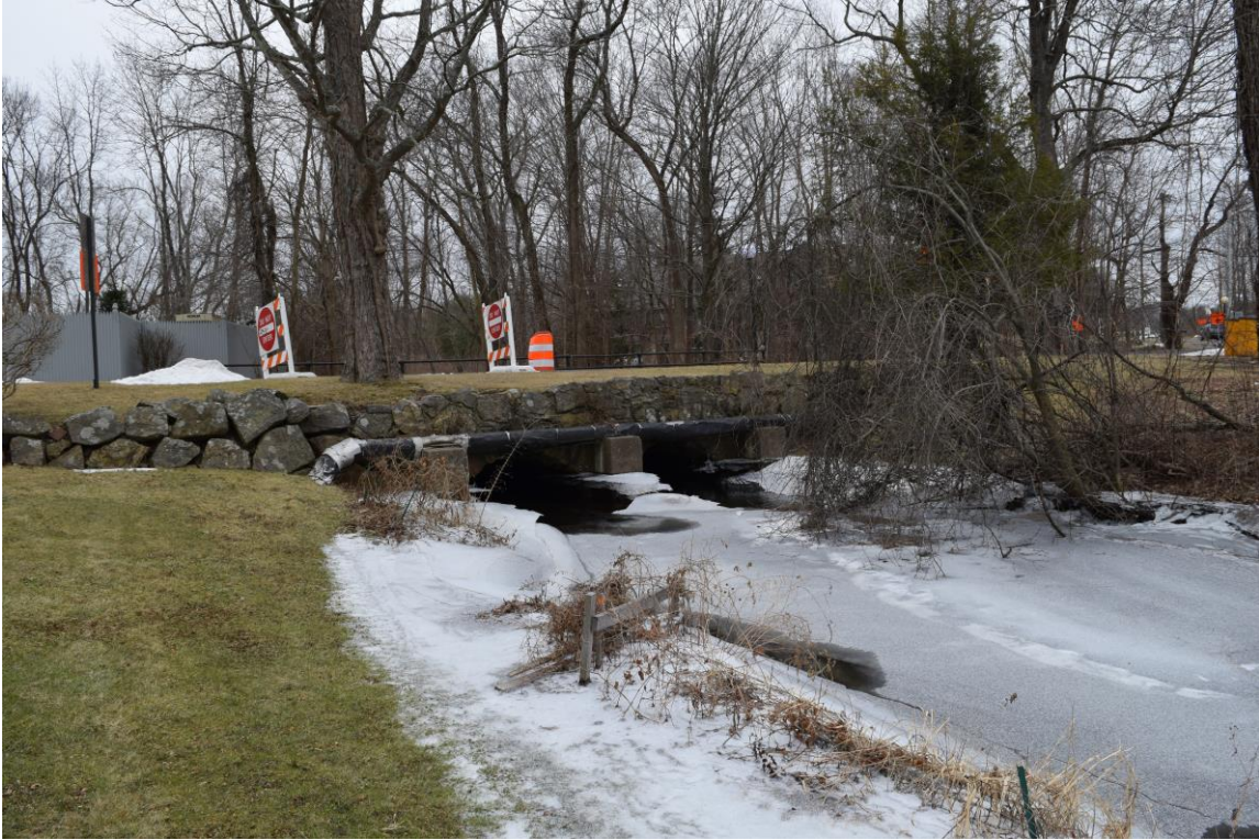
Figure 6 – Fox Hill Drive is Immediately Downstream of the Dam
