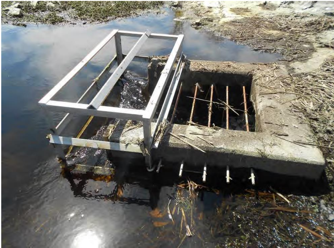
Figure 3 - Riser for Low Flow Pipe
