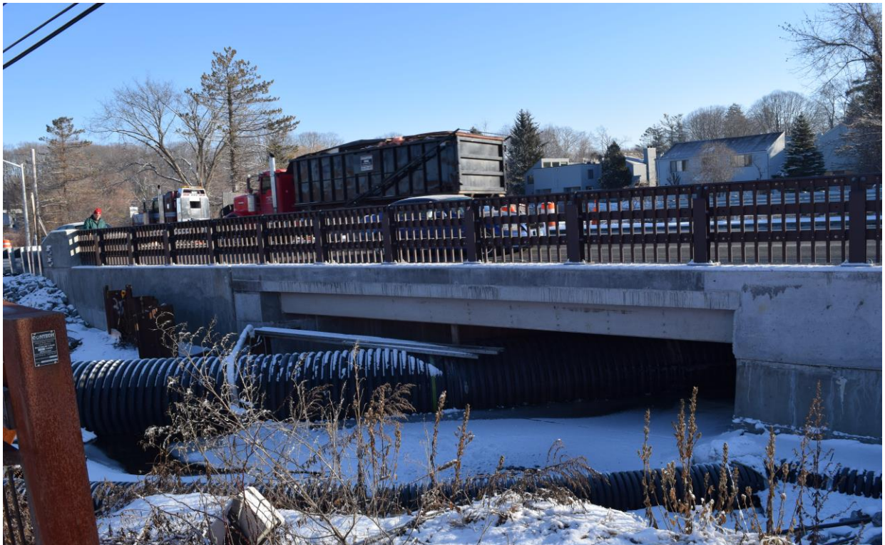
Figure 7 – Route 35 (Danbury Road) Bridge is Downstream of the Dam
