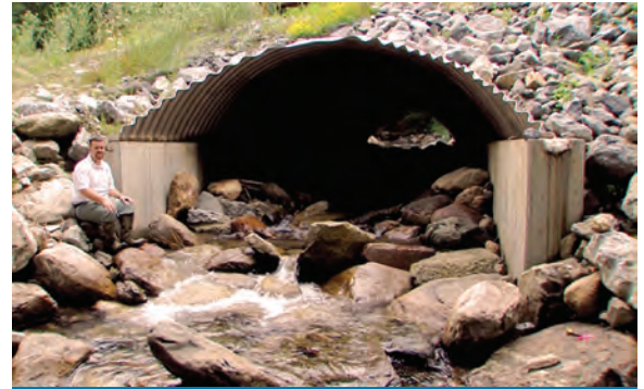
Infrastructure Project and Natural Systems Protection: This reconstructed culvert in Moosalamoo National Recreation Area in Arlington, Vermont uses rocks and sand to simulate a natural fish passage.
