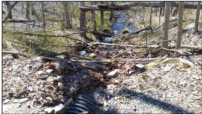
Wetland #11 – Culvert and unnamed stream along utility easement
