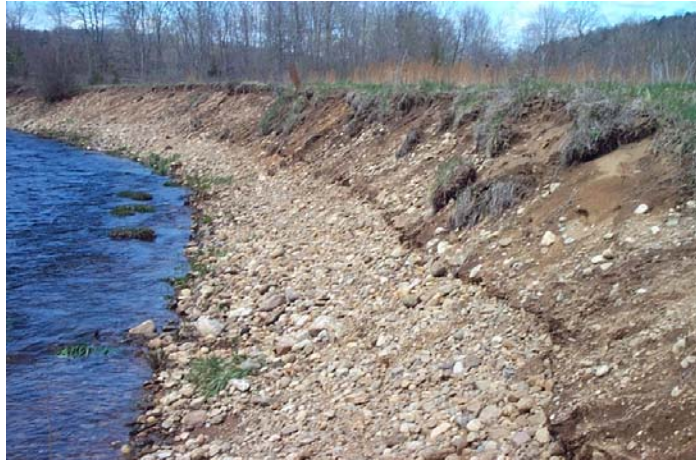
Streambank Erosion Before Restoration
