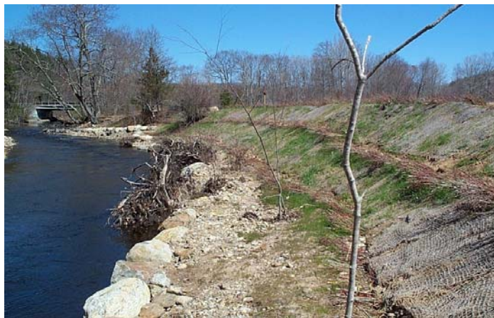
Streambank After Restoration
