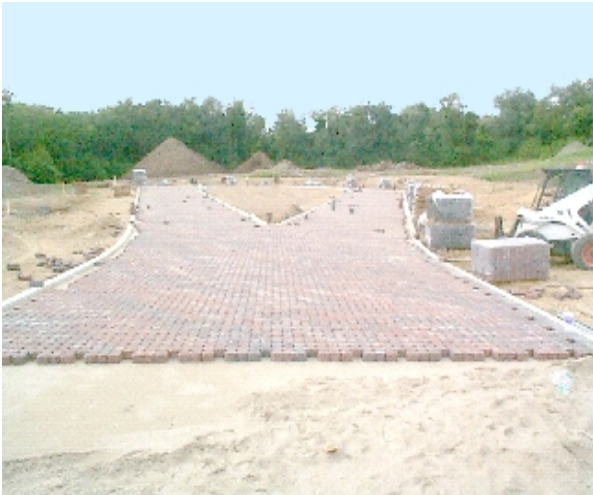
Installation of pervious pavers at the Jordan Cove national Monitoring Project site in Waterford
