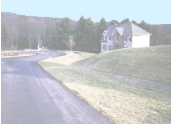
Engineered grass swale used in Watertown subdivision.
