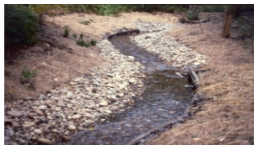
New stream channel showing lunger structures (undercut banks) and vegetative transplants
