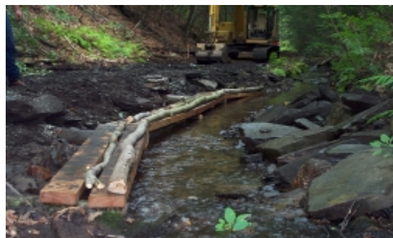
Construction of lunkers simulating undercut banks
