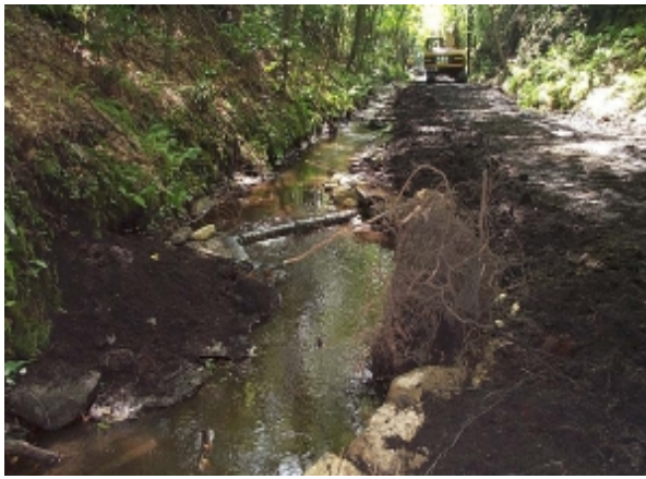
Cross - log and rootward revetment with point bar
