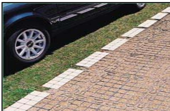
Figure 4.12 – Permeable pavement. Source: Connecticut, 2004.
