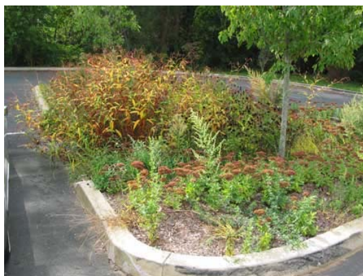
Figure 4.10 – Bioretention in use as a parking lot island in Branford, CT. Source: Connecticut Department of Environmental Protection.
