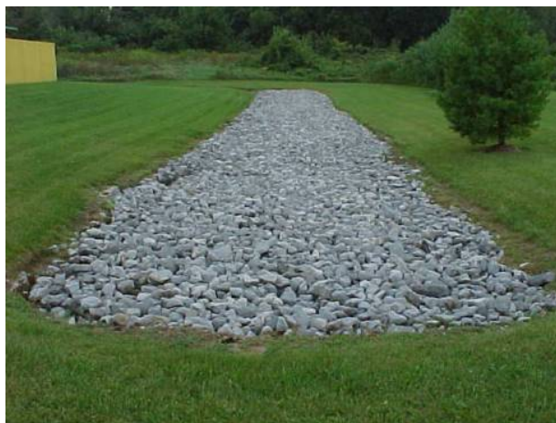
Figure 4.24 – Infiltration trench.
