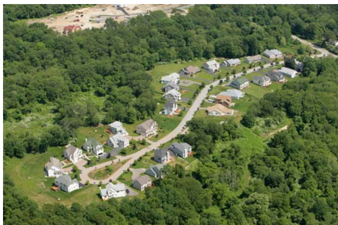
Figure 4.3– Alternative roadway design in Waterford, CT. Source: Tom Walsh, Shoreline Aerial Photography
