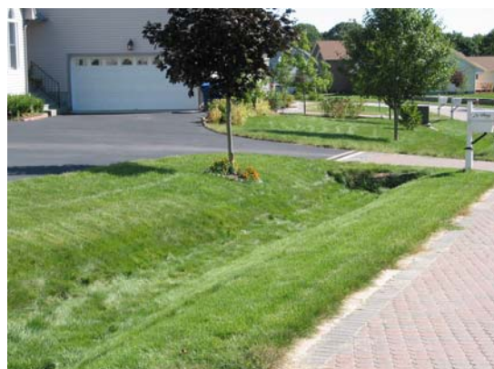
Figures 4.16 – Vegetated drainage way. Photograph courtesy of the University of Connecticut NEMO program, Kara Bonsack
