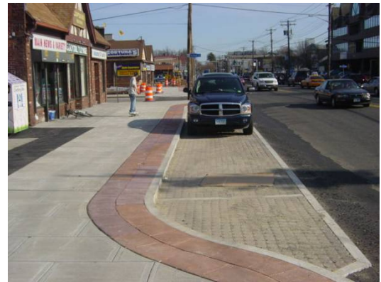
Roads are narrowed and permeable pavement is installed along roadways to provide additional parking and treat runoff.
