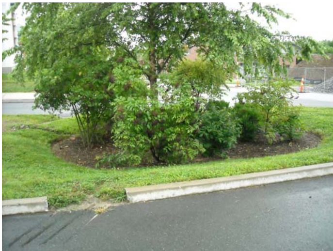
Figure 4.22 – Bioretention at University of Connecticut Storrs Campus –Mansfield, CT. Source: Connecticut Department of Environmental Protection.
