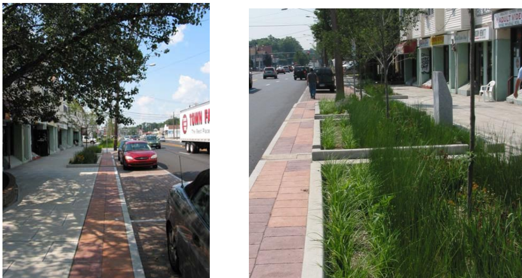
Figure 3.12 – Permeable pavement (left photograph) and rain garden/bioretention (right photograph) retrofits along North Main Street in Bridgeport, CT.
