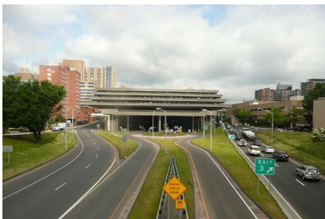
Figure 4.9 – Parking deck – New Haven,
