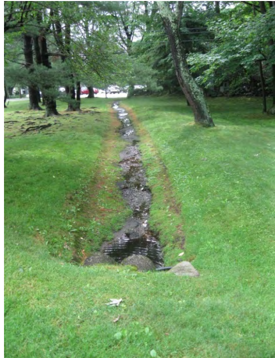
An existing swale identified for potential retrofit to improve stormwater management capability and reduce erosion.
