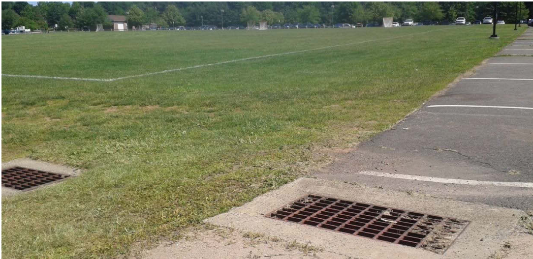
Figure 23. Existing catch basins at the edge of the swimming pool parking lot at Bartlem Recreation Area. The space between the parking lot and ball field is proposed for conversion to a vegetated swale.
