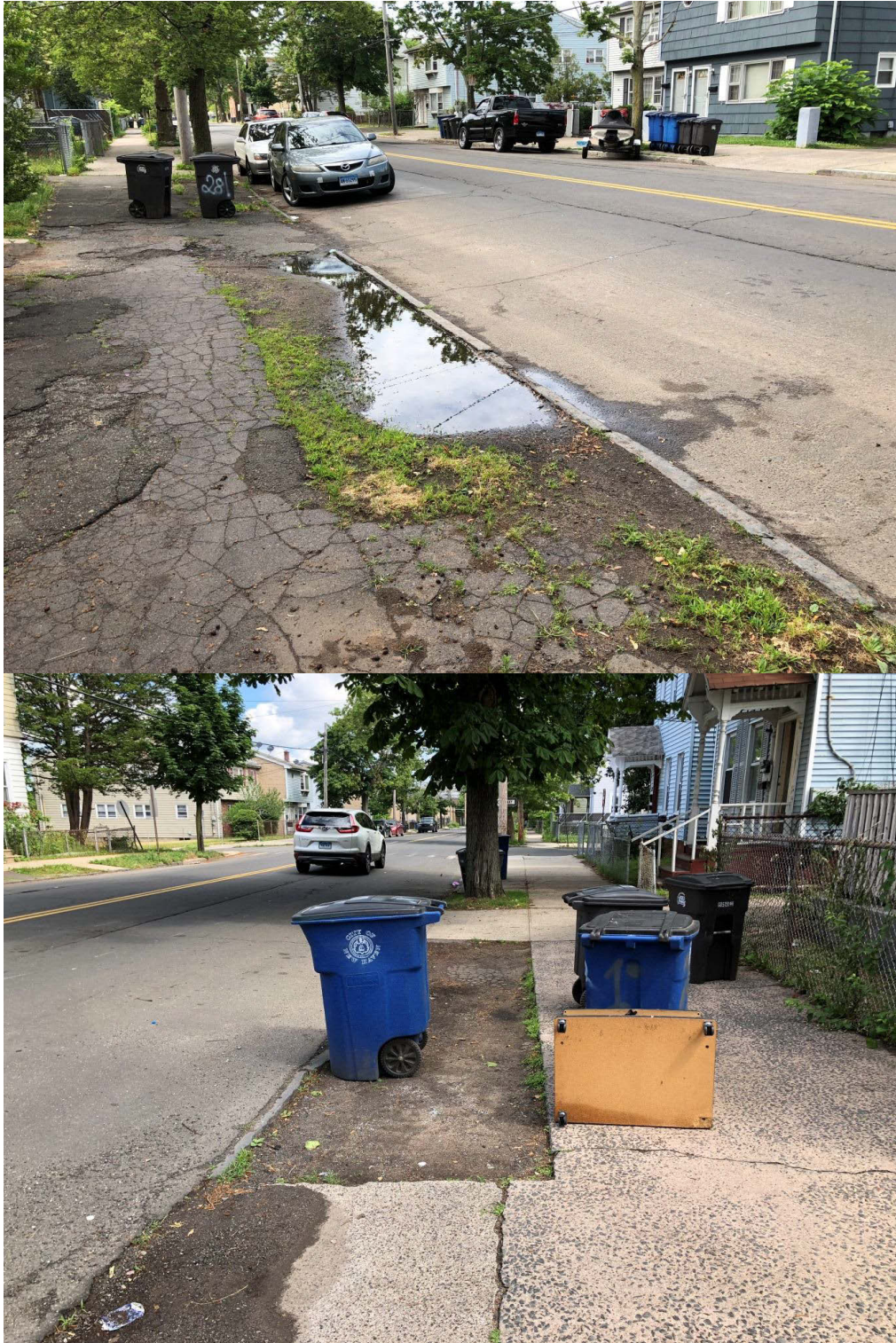
Figure 7. Existing conditions along James Street, New Haven highlighting possible locations for bioretention practices in the right of way along James Street.
