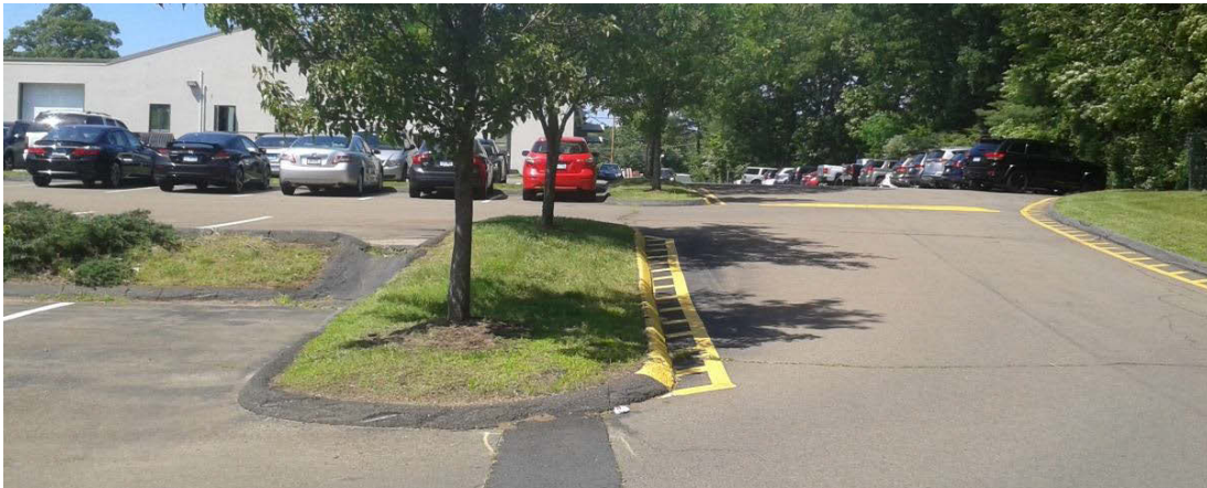
Figure 16. Tiered parking, with existing conveyances that transport stormwater from the upper tiers to lower tiers.
