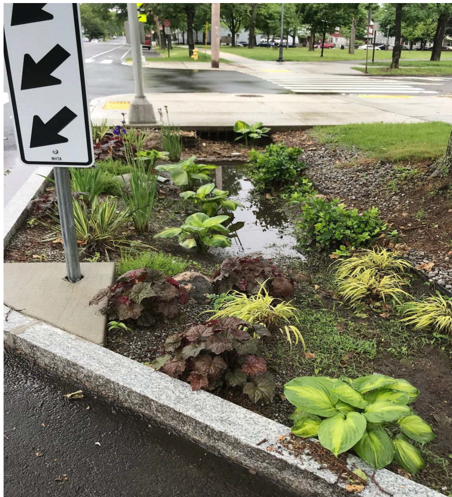
Figure 9. (above) Bioswale installed in the City of New Haven. Credit: Dawn Henning, City of New Haven Engineering
