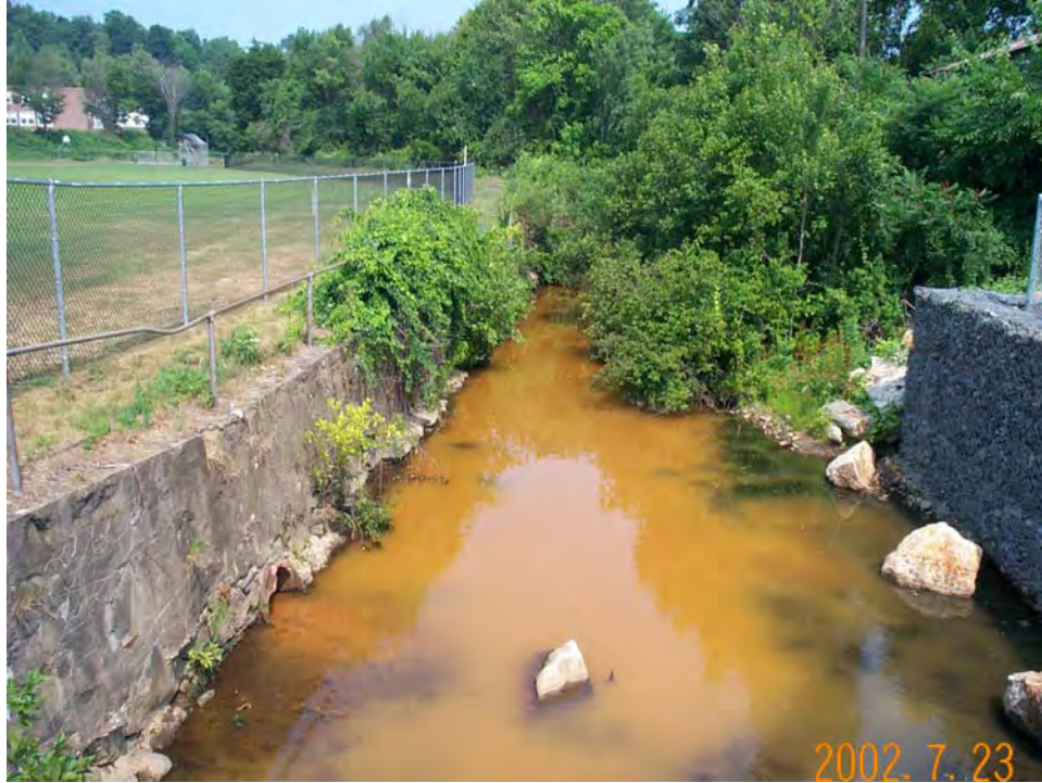
Figure 8: Steele Brook downstream of dam exhibiting high orange discoloration. (Photograph courtesy of CT DEP)
