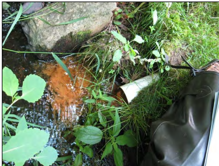
Outfall pipe originating from a residential property on the left bank of segment TB-04C.
