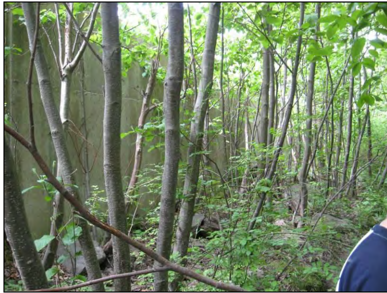
Concrete retaining wall adjacent to Gerber Drive along segment GB-03B
