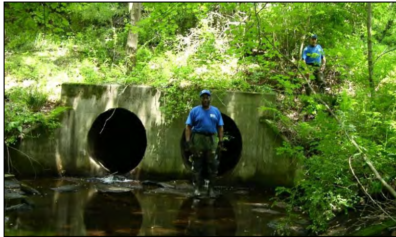
Bamforth Road crossing (perched culvert) along reach CB-03
