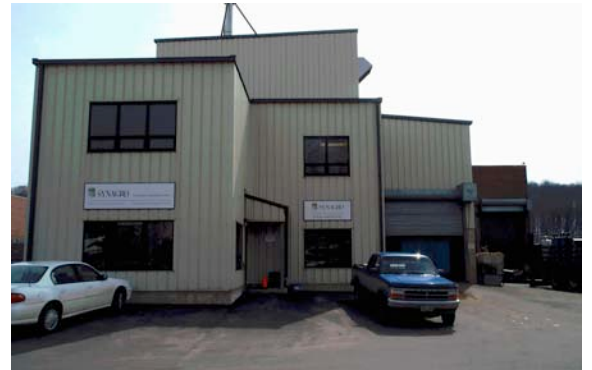
Synagro Incinerator in Waterbury (FOG used as a Supplemental Fuel Source)
