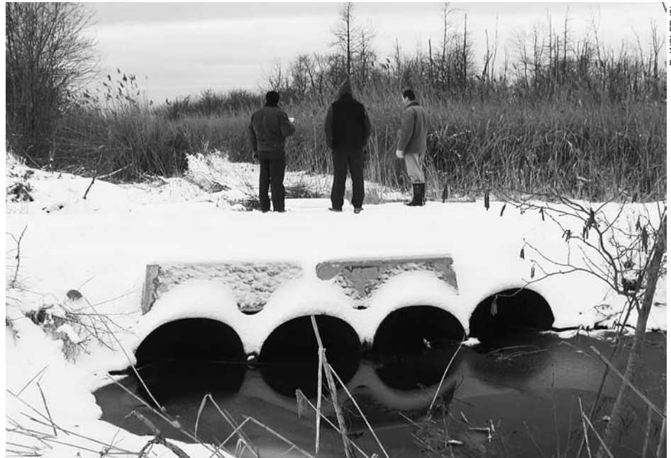
The WHAMM Program worked with the City of East Haven to install culverts and excavate channels to restore tidal flow to a marsh.
