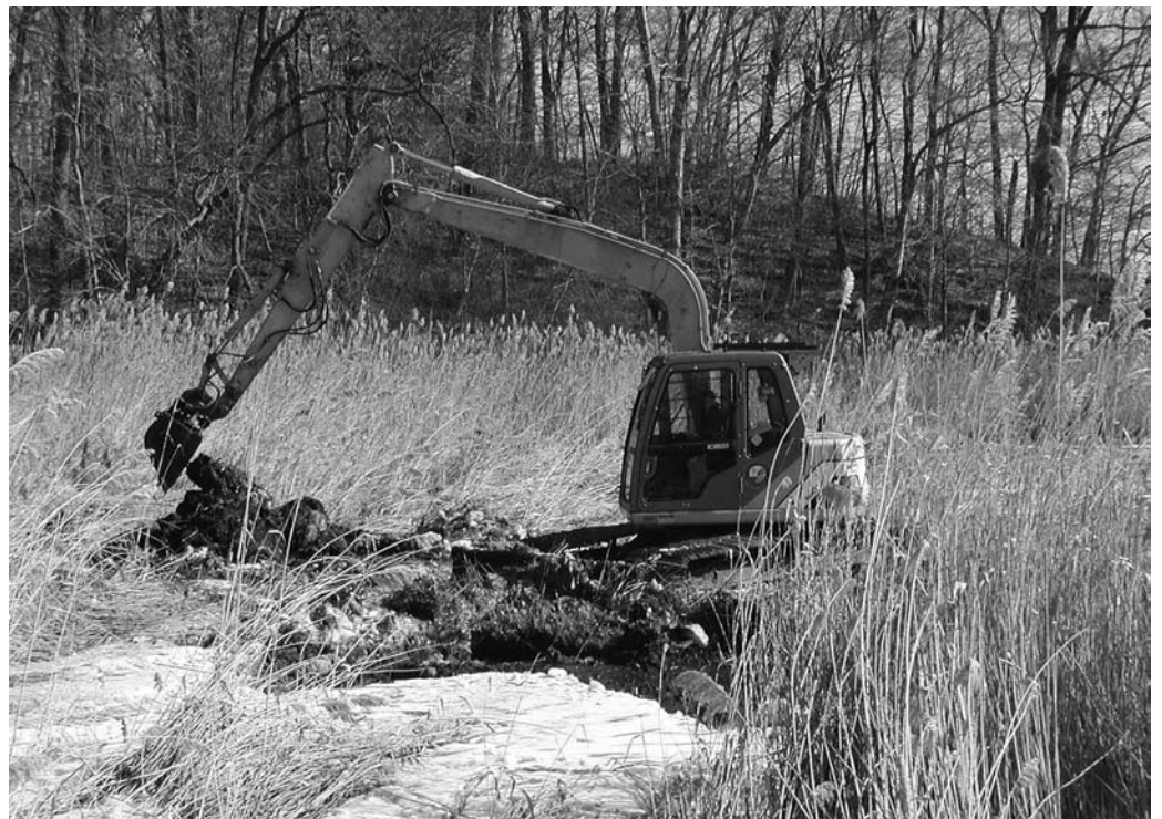
A wide-tracked excavator creates shallow pools and channels to eliminate mosquito breeding and enhance wildlife habitat.
