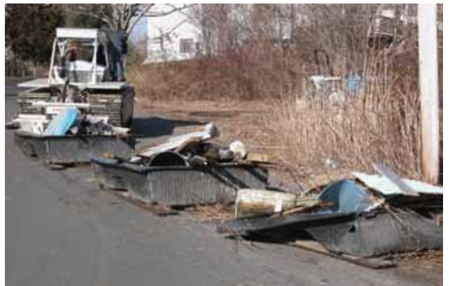
Several sleds can be chained together to increase the efficiency of debris removal.
