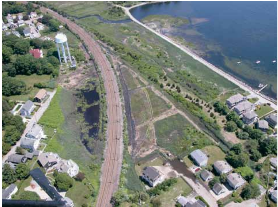
The Stonington Borough marshes can be seen north and south of the railroad tracks. This photograph shows the newly cleaned ditches in the marsh to the south. The marsh to the north was not yet completed when this photograph was taken on June 8, 2012.
