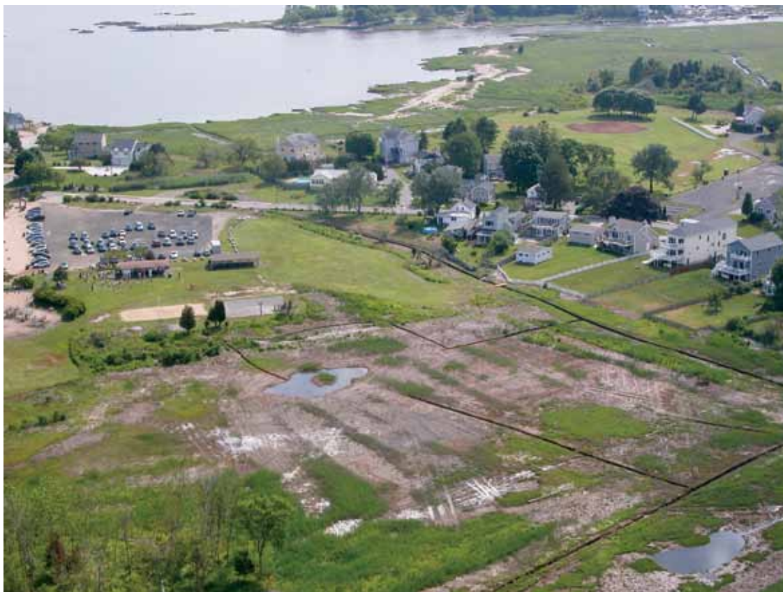
A view of the wetland restoration work conducted at Jacob's Beach off of Seaside Avenue in Guilford. Note that several pools and linear channels have been cleaned. This photograph was taken on June 14, 2012.
