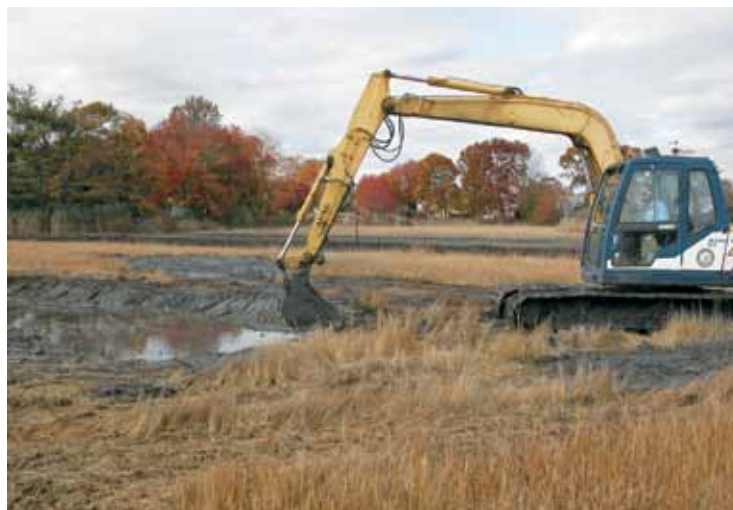
A low ground pressure (less than three pounds per square inch) excavator is used on soft marsh soils to create shallow pools and channels to enhance fish and water bird habitat and control mosquitoes.
