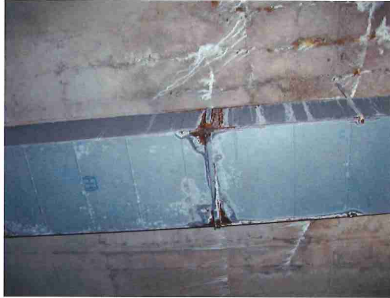
PHOTO 2 Parking Level P3
