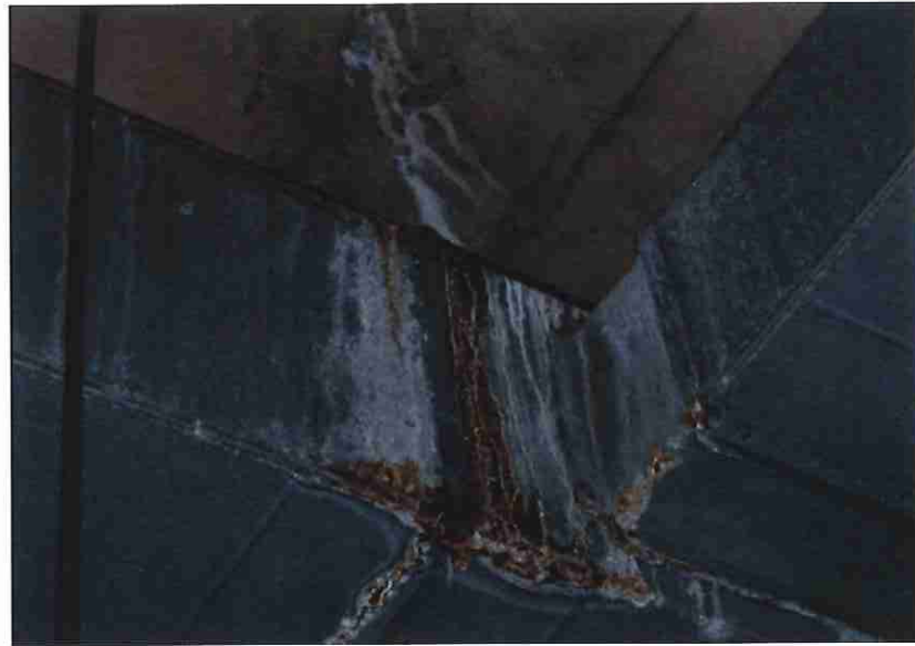
PHOTO 1 Parking Level P3
