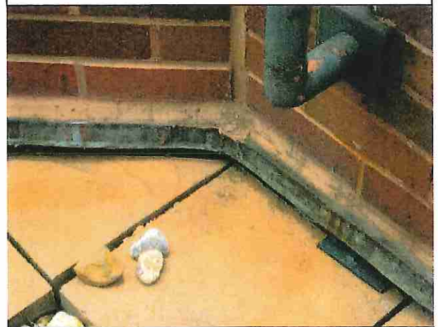
Sealant Covering Weep Holes
