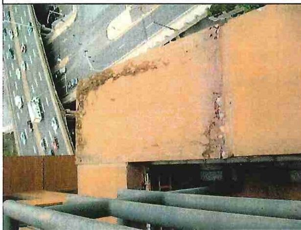
Cracking Capstone
