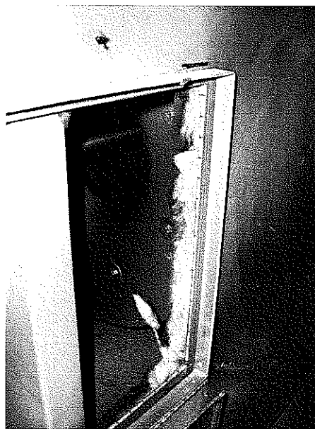
Figure 1 - Air handling unit with failing insulation
