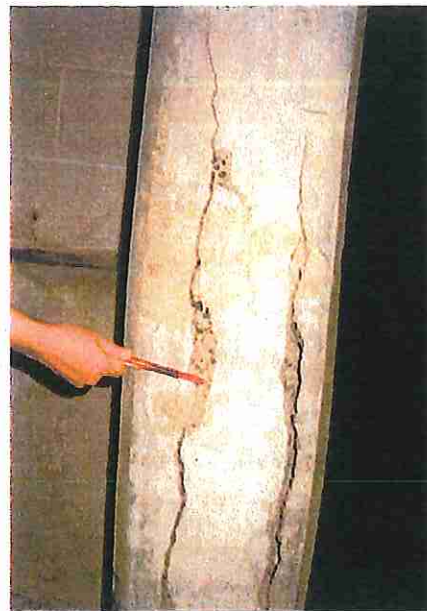
Photo 9: Drawings indicate this area is transitioning from 14 vertical bars to 16 bars; the 16 bars extend up from the floor below to provide a lap splice with 14 bars coming down from above.
