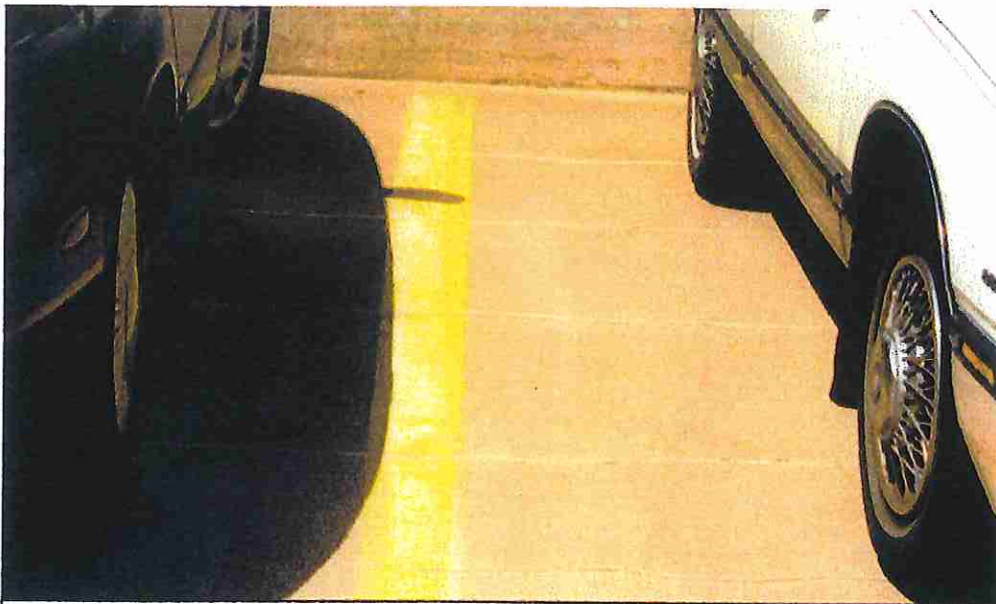
Photo 18 -Again at roof but over cantilevered section of beam. (parapet is in background)
