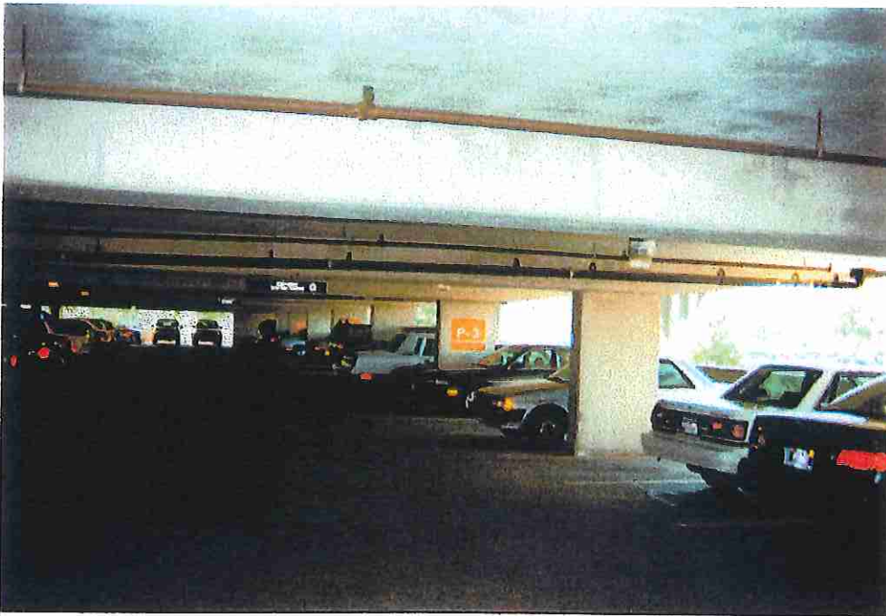
Photo 22: Looking west through cantilevered and post tensioned garage structure.
