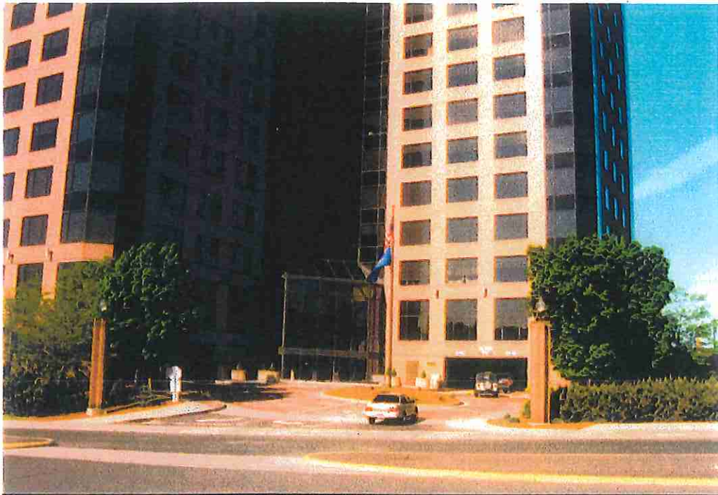
Photo 1: Exit (on left) and entrance (on right) on the east elevation. Garage extends under circular plaza area.
