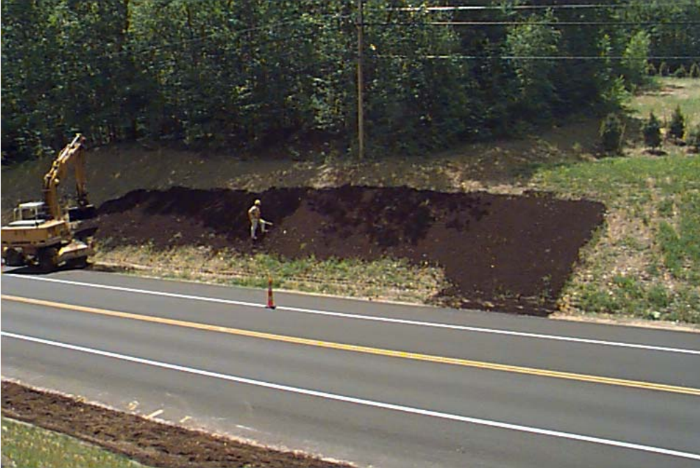
Photo #2. Extra Compost Being Placed on 2:1 “Dead Sand” Slope Near Station 267+50
