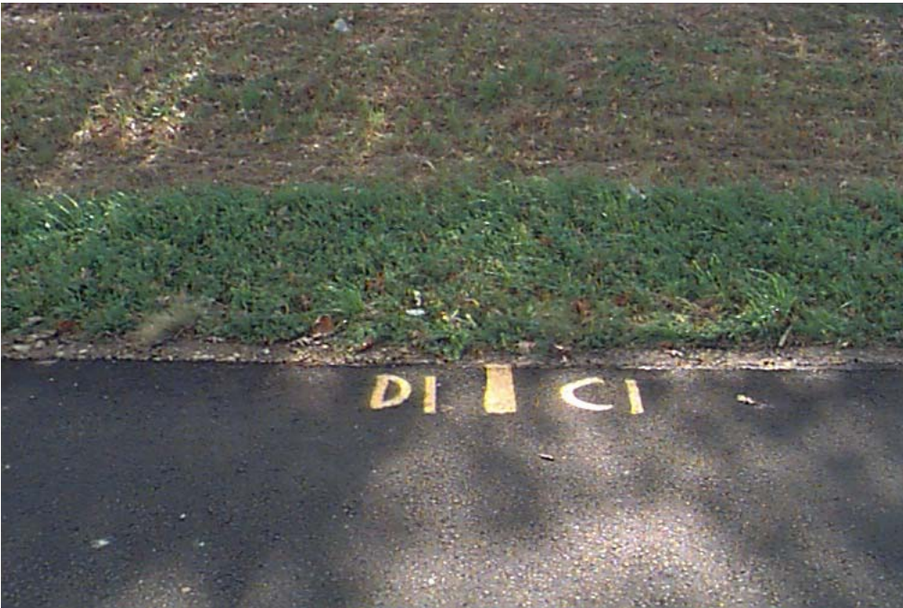
Photo #16. Interface of 1/2 Inch and 1 Inch Compost Sections (October 19, 1998)
