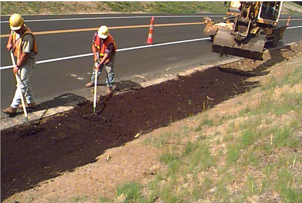
Photo #7. Spreading the Compost at Section C2
