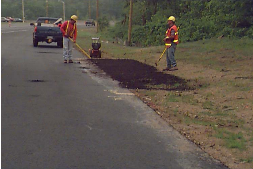
Photo #4. Spreading the Compost for Top Dressing onto Section E1 (station 124+18)
