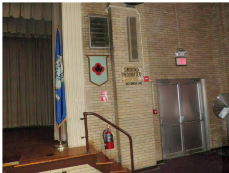
Egress door in auditorium
