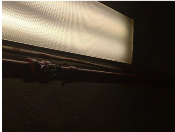
Surface mounted fluorescent fixture
