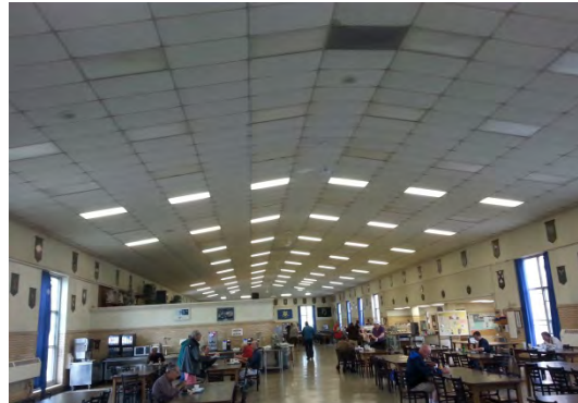
Recessed fluorescent fixtures in the dining hall
