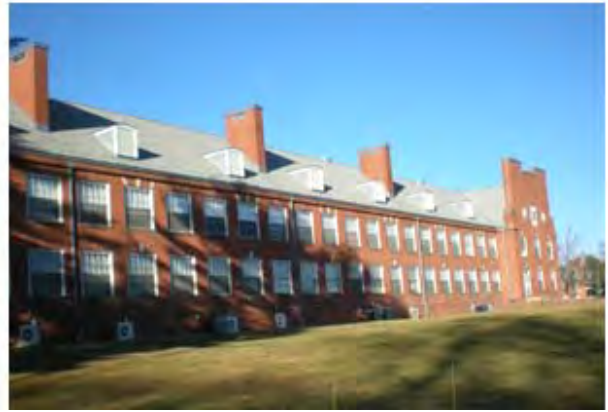
Southwesterly Wing of Building #3
