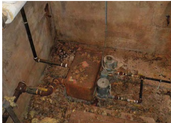
Electric Condensate Pump
