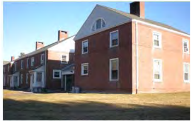
Northwesterly Corner of Building #51
