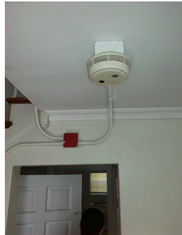
Typical smoke detector
