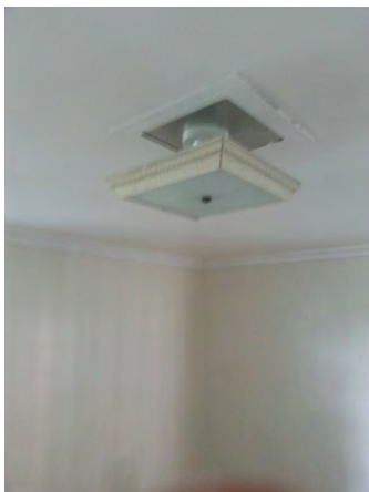
Typical fixture part of original construction
