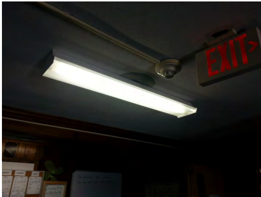
Typical fluorescent fixture
