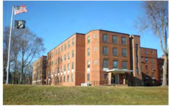
Southwesterly Wing of Four Story Building – Northwesterly Wing of Five story Building
