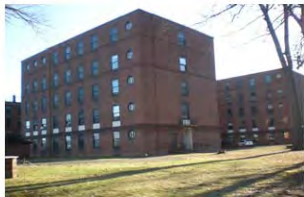
Northwesterly Wing of Five Story – Built 1945
