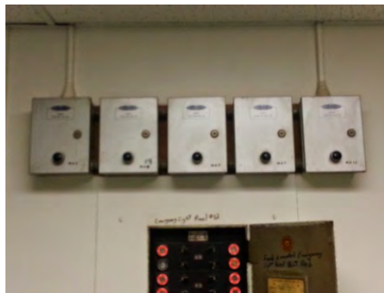
Dual-Lite relays for emergency lighting
