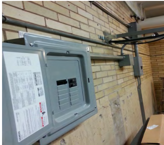
125A-1Ø panel feeding head-end equipment
