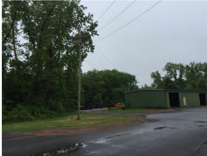
24kV Power Lines from street
