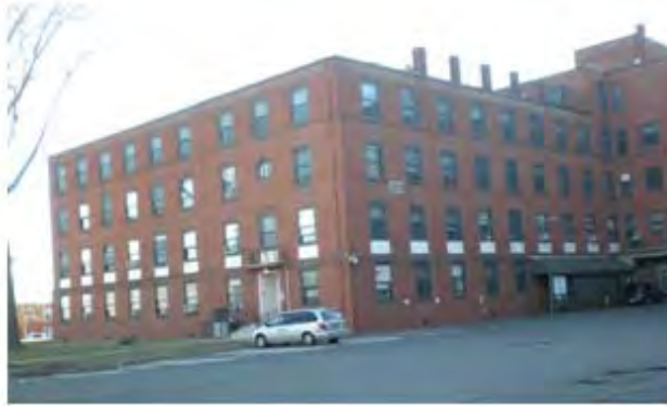
Easterly Wing of Four Story – Original Building
