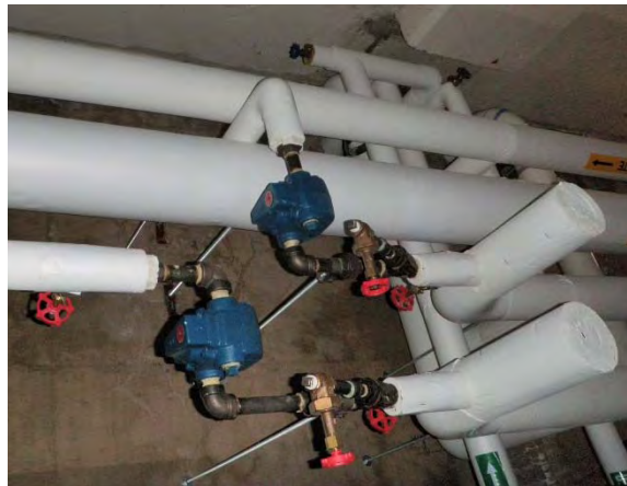
New steam traps and condensate piping connecting to existing main
