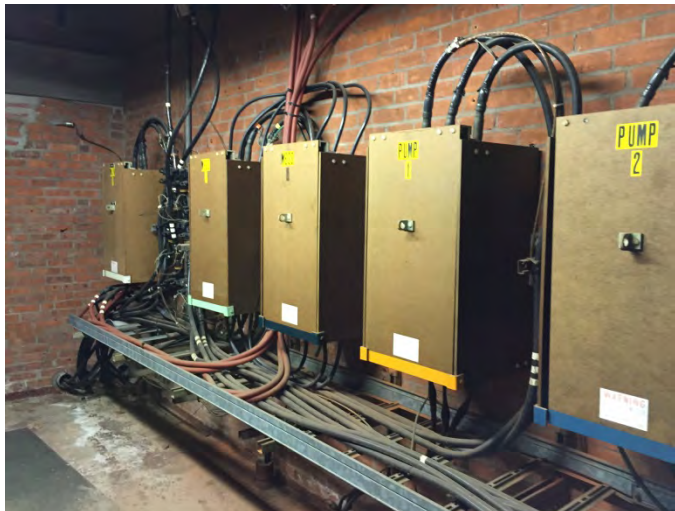
Fused feed-throughs for six distribution lines
