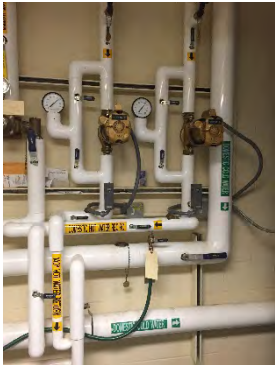
Domestic hot water distribution system
