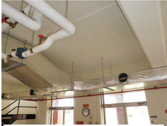
Ducted DX split systems without diffusers
