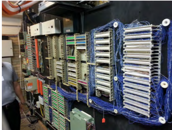
Telephone punchdown blocks
