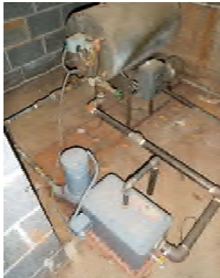
Electric Condensate Pump
