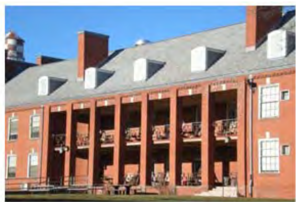
Westerly End of Building #4
