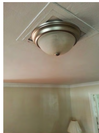
Typical renovated fixture
