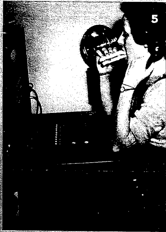
TWENTY HOURS A DAY during the emergency this clerk at Essex remained at the switchboard.
