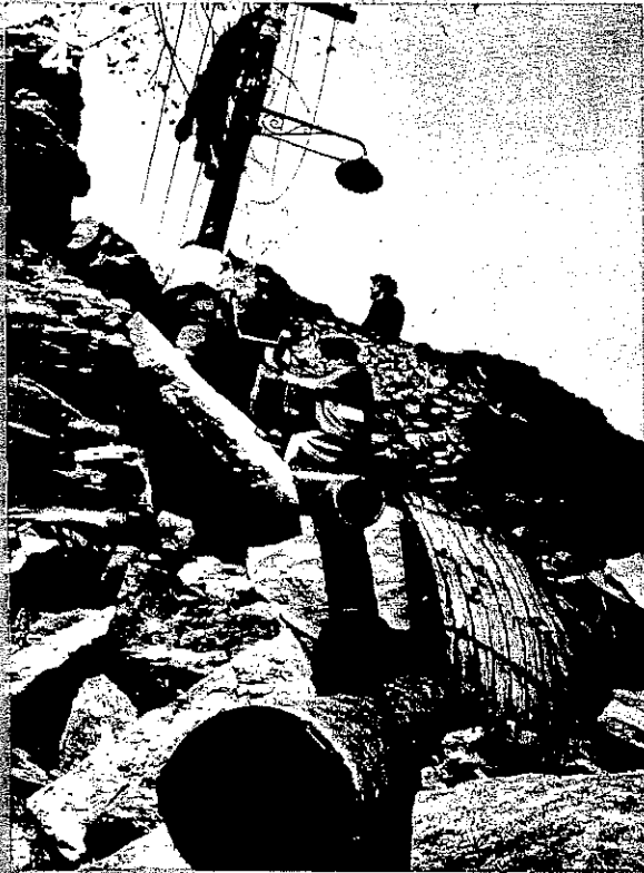
DISRUPTED were electric, gas and water services in Rockville. Company men are repairing two.
