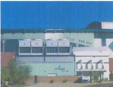
NRG Energy Center Phoenix District Energy Plant
