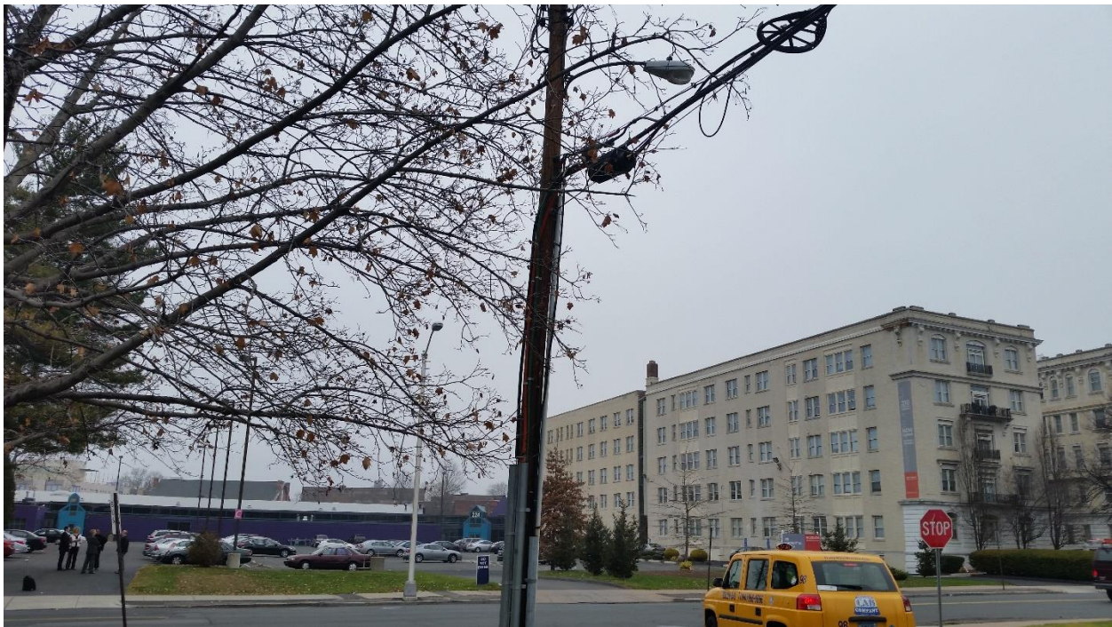
Figure 2: Conference of Churches – Comcast Fiber Stored Directly Across Street
