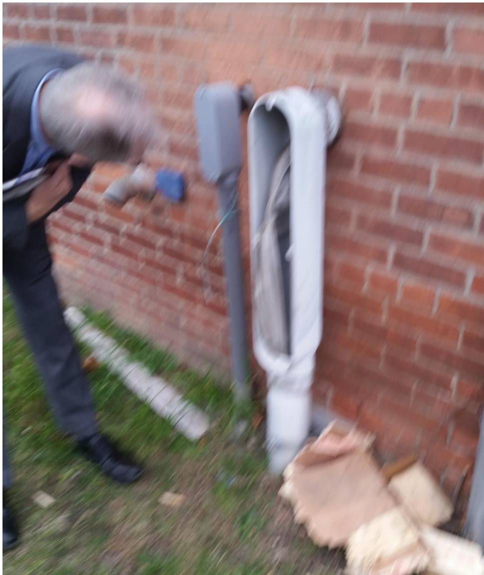
Figure 5: Scotts' Jamaican Bakery – Fiber Terminated at Warehouse Across Street
