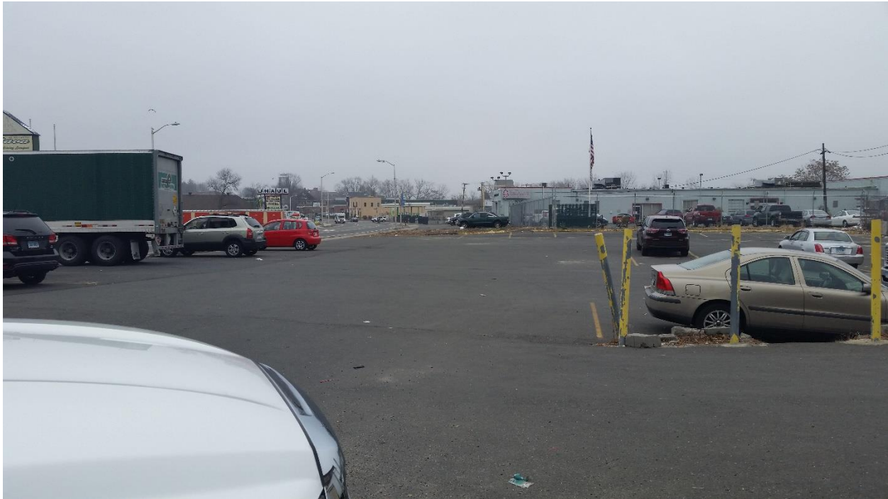
Figure 9: Express Kitchens – View Across Parking Lot Where the Business Constructed Conduit
