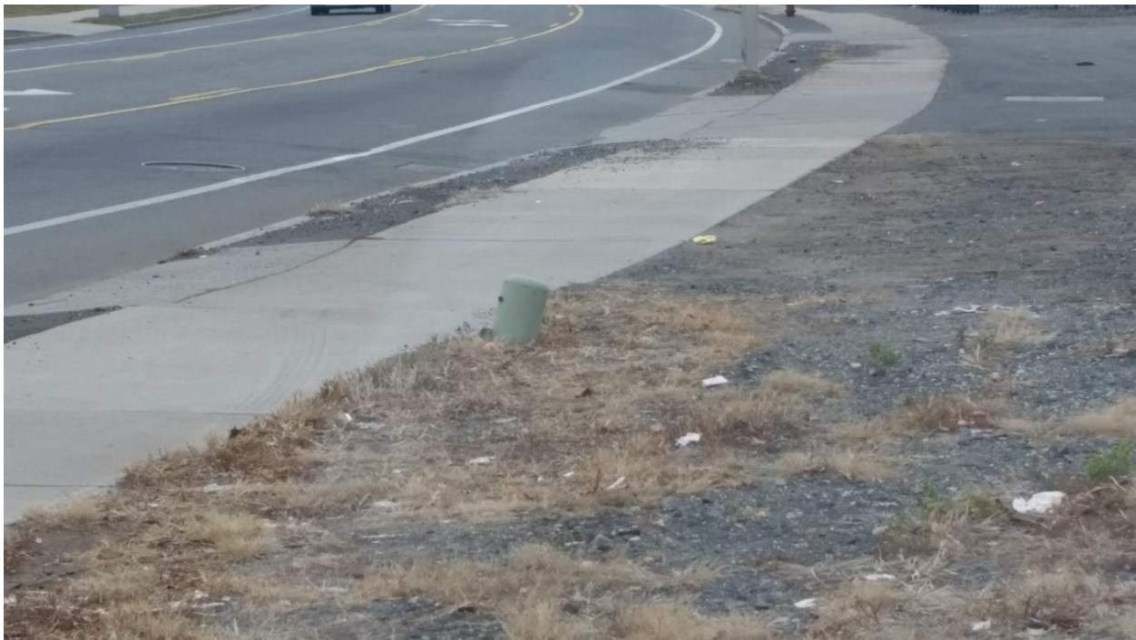
Figure 8: Express Kitchens – Pedestal on Adjacent Vacant Residential Lot
